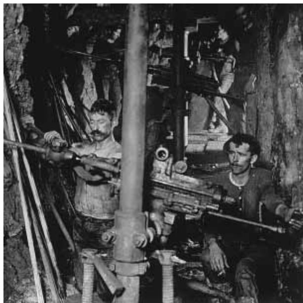
Figure 19–1 In the early 1900s, miners extracted gold, copper, and other metals from underground mines such as this one 600 meters below the surface in Butte, Montana. (Montana Historical Society)
