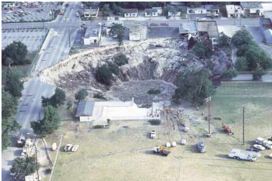
Figure 15-20 This sinkhole in Winter Park, Florida, collapsed suddenly in May 1981, swallowing several houses and a Porsche agency. (AP/Wide World Photos)
