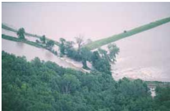
Figure 14–29 Flood waters pouring from the channel of the Missouri River through a broken levee onto the flood plain in Boone County, Missouri. (Stephen Levin)
