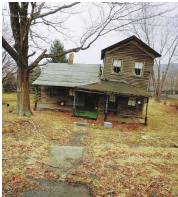
Figure 19–16 This house is being torn in half and tilted as it sinks into an abandoned underground coal mine. (Chuck Meyers/U.S. Department of the Interior)
