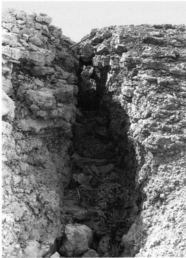
Plate 12.10 Close-up of partially collapsed pipe of Plate 12.9 . (Photograph: Vita-Finzi, 1985)
