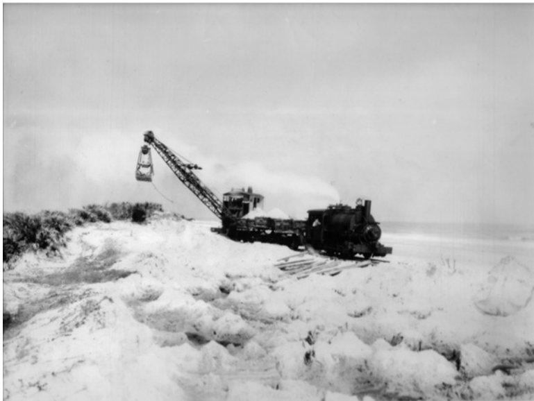
Frontispiece B. Mining in 1919 on the beach at Mineral City, site of the current Ponte Vedra Beach ~24 km southeast of Jacksonville, FL. This is the first heavy-mineral sand mining operation for titanium minerals in the USA. Mining was done by the clam-shell at the end of the train. The locomotive transported the ore in the cars to a wet mill over a narrow gage wooden track. The mill was adjacent to the beach. Photograph courtesy of the Beaches Area Historical Society, Jacksonville Beach, FL.
