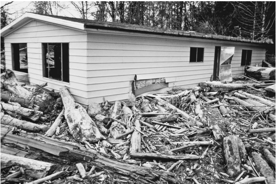
Devastation along the South Fork Toutle River resulting from the May 18, 1980, lahars. Logs and other debris jammed up against the house. (Lyn Topinka, USGS)
