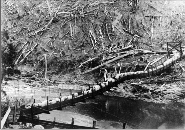
Figure 7.9 River responses to forest clearance on the North Eastern Cape of North Island, New Zealand Rapid clearance of forest cover and the introduction of sheep brought about dramatic adjustments to river character and behavior, as indicated by bank erosion on this photograph taken immediately following the impact of Europeans in this part of New Zealand. Photograph titled "Sheep crossing Mata River, East Coast, New Zealand, Puketoro Station" by Frederick Hargreaves. Reproduced with permission from the Tairāwhiti Museum, Gisborne, New Zealand.
