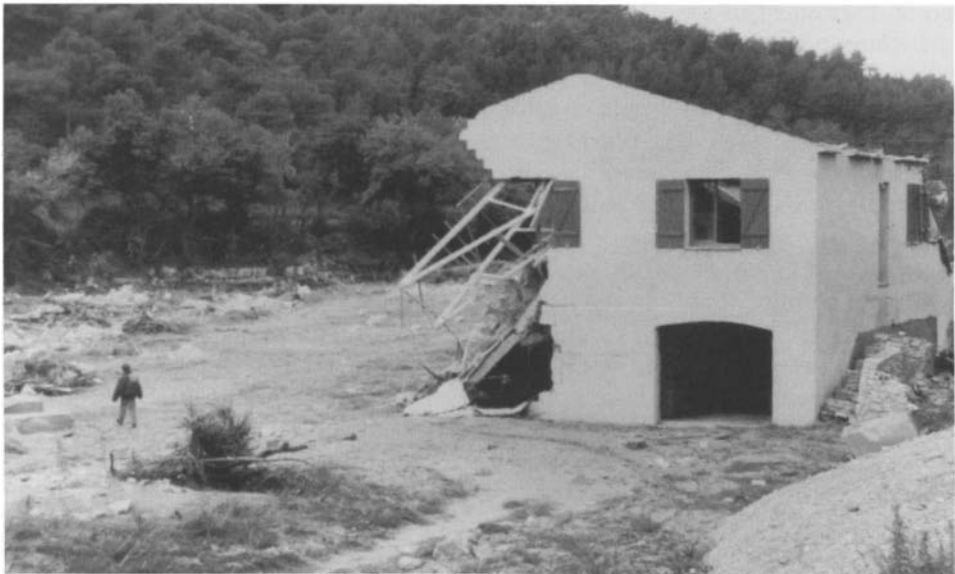
Fig.6.3 A ( upper ): The floodplain of the Ouvèze, looking upstream from Vaison, after the flood of 22 September 1992 (most debris has been removed); B ( lower ): Destruction of a house by the same flood (J-P.Bravard)
