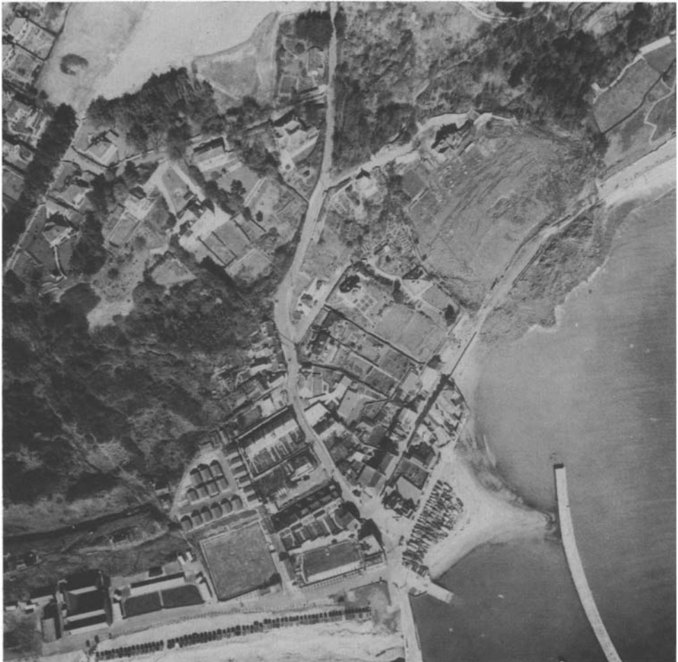
Fig.8.7. The Cliff House landslide at Lyme Regis, 1962. Vegetated and degraded cliffs in Liassic clay can be traced across the photo, which over time have been developed for housing, especially where the Cobb Road descends the cliff. During the slide, Cliff House was destroyed, but the shear surface did not displace the esplanade.
