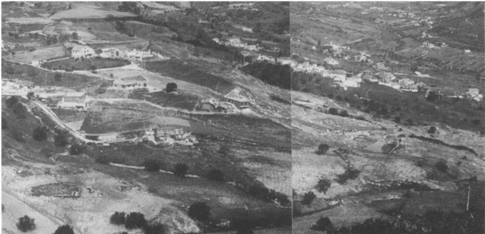
Fig.16.8. The road along the Trancão valley was washed out during the 1983 flash flood in the Lisbon region (photo: A.de Brum Ferreira).
