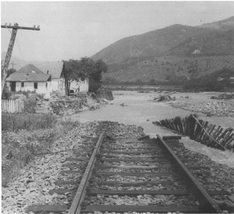
Fig.17.6. Destruction of the Buzău-Nehoiș railway in June 1969 by flooding on the Buzău river at Păltineni (Photo: D.Bălțeanu)
