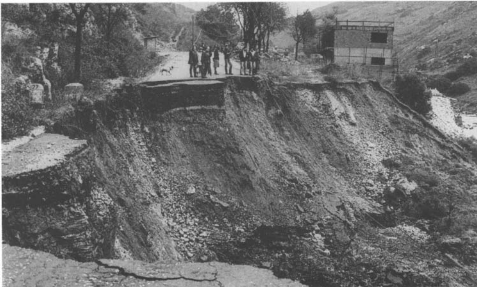
Fig.16.7. The Calhandriz landslide that occurred north of Lisbon, in February 1979, destroyed several houses, some of them newly built (photo: A.de Brum Ferreira)
