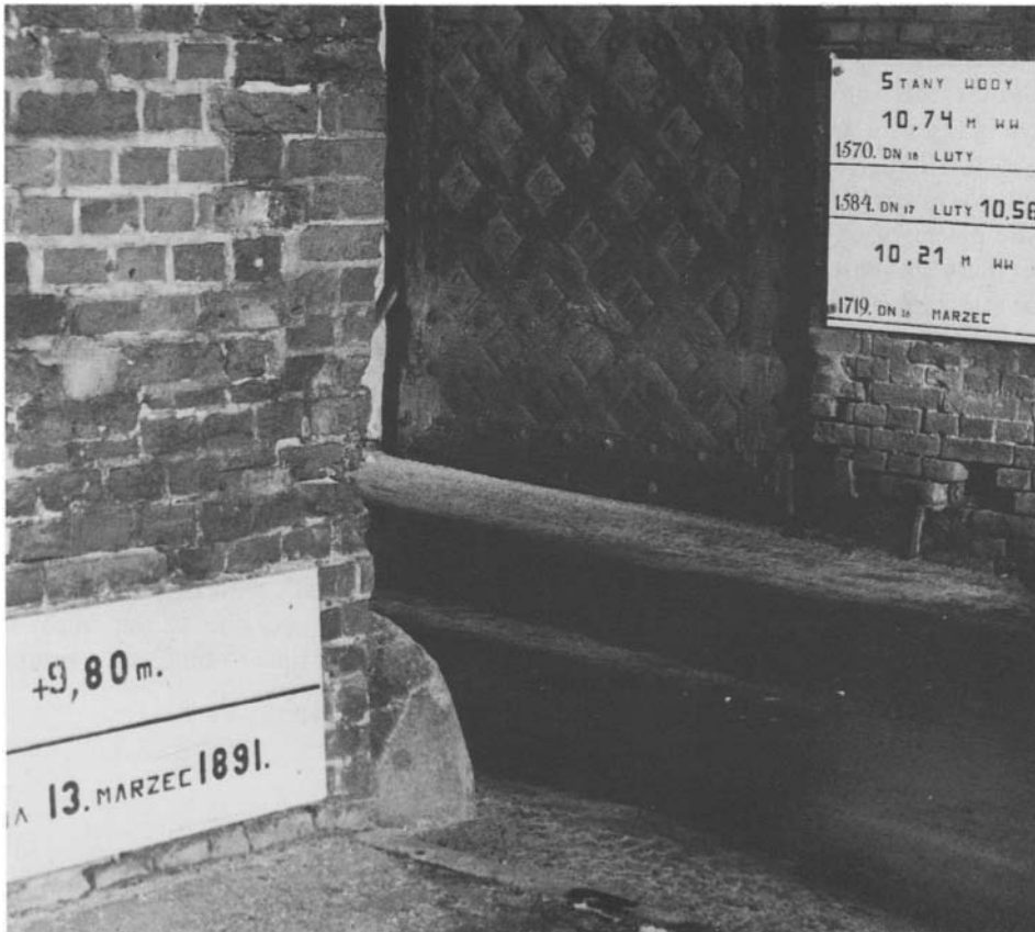
Fig.15.1 High-water marks on the walls of the old city in Toruń (photo M. Grześ)
