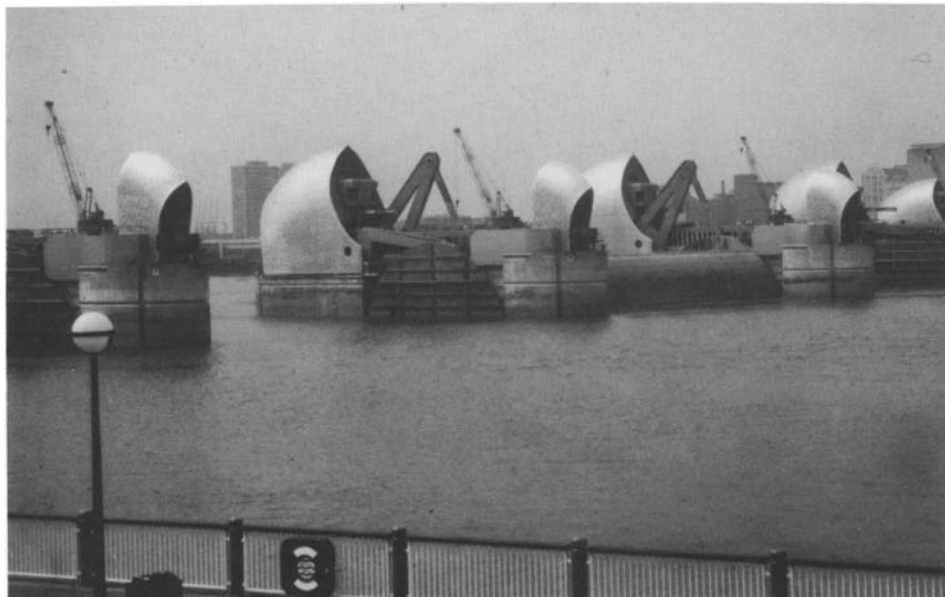
Fig.8.11. The Thames Flood Barrier, Woolwich. One of the gates (to the right of centre) is partially closed. (Photo: C.Embleton)
