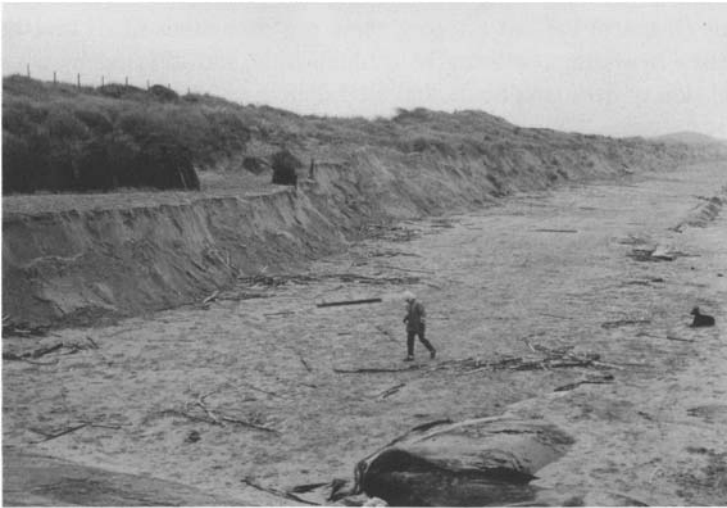
Fig.2.11. Formation of a beach cliff and erosion of the coastal dune belt by a storm surge in the autumn of 1993 (Photo: I.Heyse)
