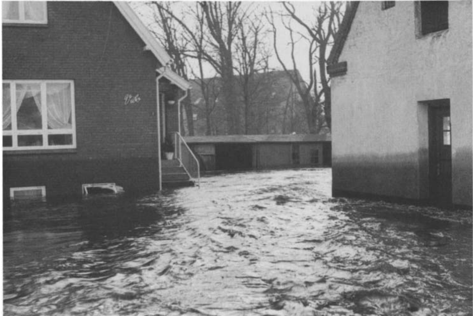
Fig.4.5. Flooding in Holstebro in March 1970. The high-water mark can be clearly seen on the wall of the house to the right. The basement of the house was filled with water-transported sand. Large parts of this town, which had never suffered from flooding before, were badly damaged and the people had to be evacuated.
