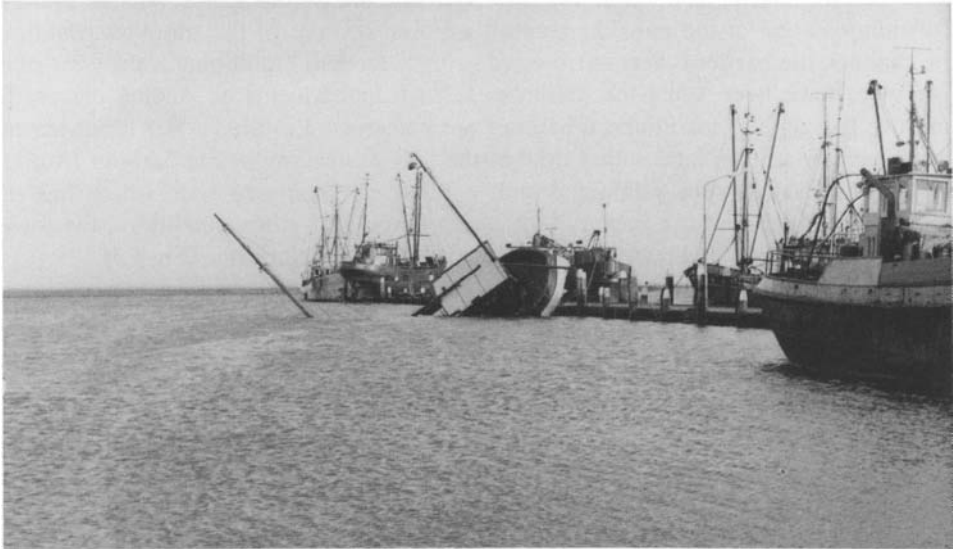
Fig.4.2. The fishing port of Rømø devastated after a storm in January 1976. In the far background, a fishing vessel can be seen dumped on the pier owing to the high water level which overtopped the white bollards. The fishing vessel in the centre foreground has its stern resting on the pier and its bows on a sunken ship. The water level is still high: normally, the decks of the ships lie below the level of the pier.
