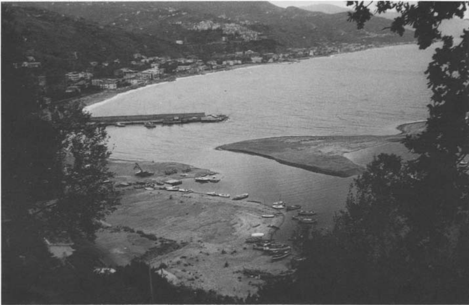
Fig.12.15. The touristic harbour of Cetraro on the Tyrrhenian coast of Calabria (1982). The small harbour is becoming silted, as a consequence of the poorly-advised construction of the jetty, in disregard of the local coastal dynamics (photo: G.Rodolfi)
