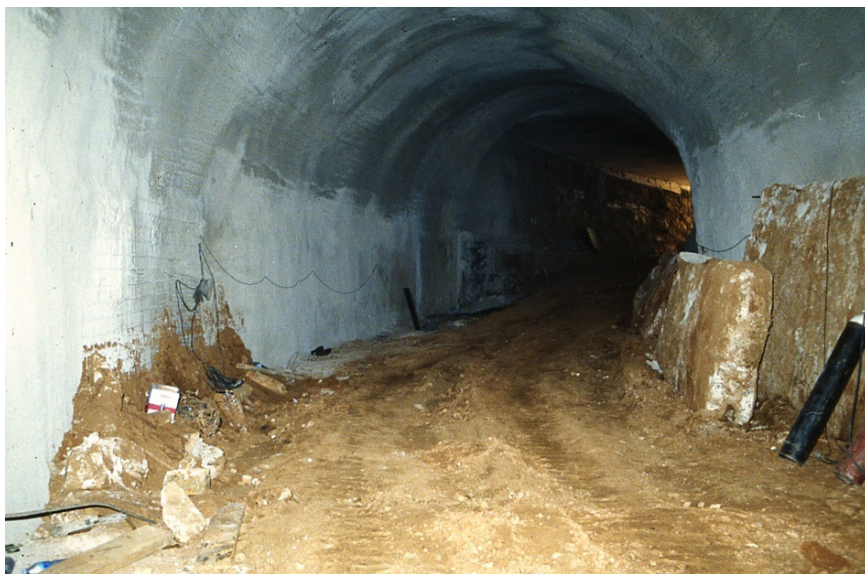
Figure 7.7 The finished tunnel.
