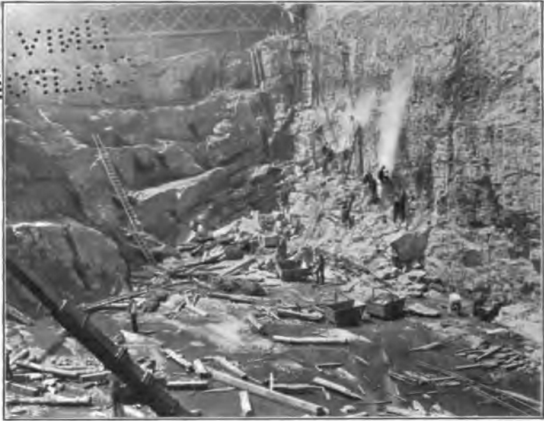
Fig. 4. Looking Southwest from 42d Street and Park Avenue Rapid Transit Excavation.
