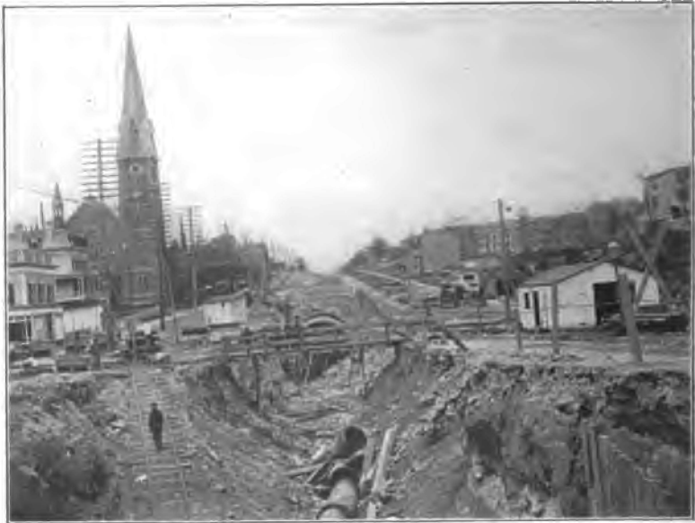
Fig. 30. Looking up Broadway through the Rapid Transit excavation from 155th Street. Heading in rock shown and partially completed arch. May, 1901.
