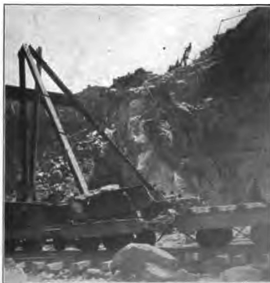
Fig. 13. Pennsylvania Railroad excavation, 32d Street, west of Ninth Avenue.
