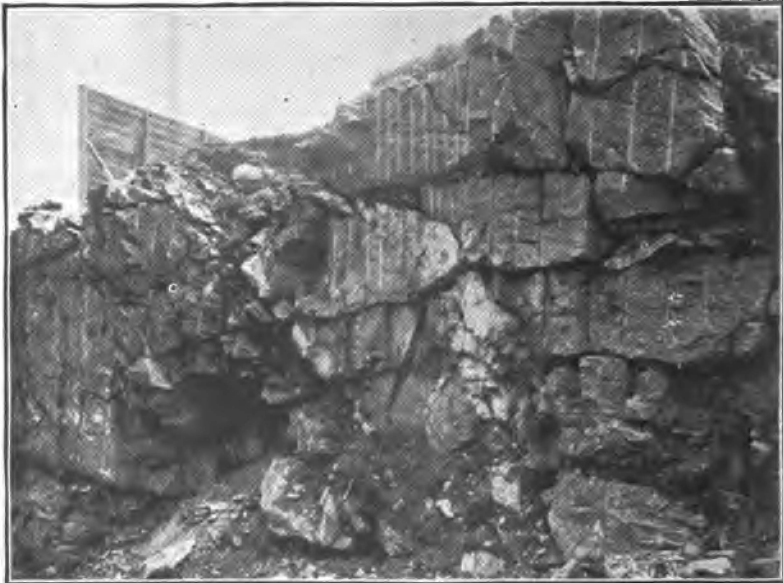
Fig. 21. South side of 110th Street, near Columbus Avenue, showing folded granite vein in very micaceous gneiss. (The vertical lines are drill holes.)
