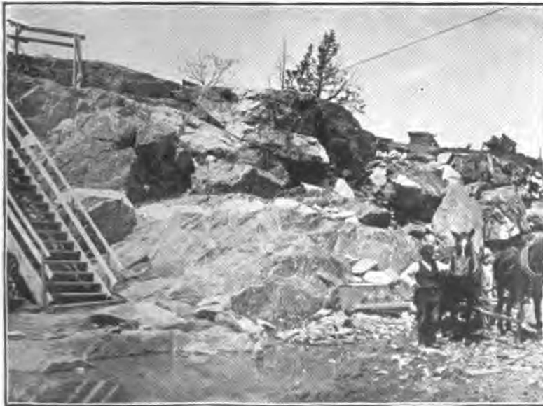
Fig. 7. Riverside Drive and 93d Street, north side, in process of removal, showing granite vein crossing quartzose gneiss.
