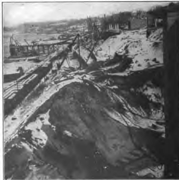
Fig. 53. Continuation of Viaduct, looking north. 1905.
