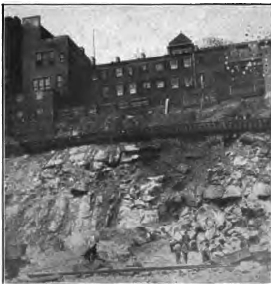
Fig. 12. Pennsylvania Railroad excavation, 33d Street, west of Ninth Avenue.
