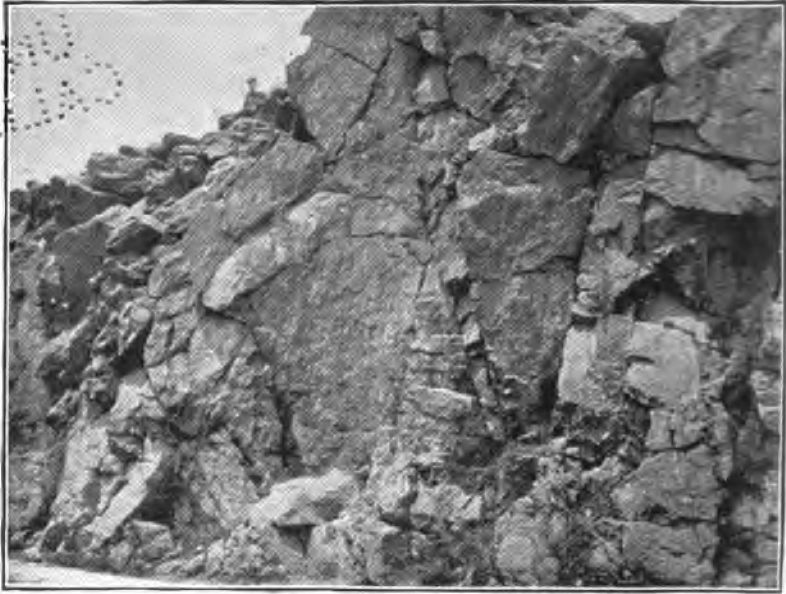
Fig. 20. North side of 126th Street, a few feet west of Manhattan Avenue, showing granite vein and shearing.
