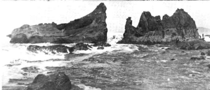
Jumpoff Joe along the coast near Newport showing erosion in 1900, 1913, and 1926. Only a small knob of the original rock remains today (photo courtesy Oregon Dept. Geology and Mineral Industries).
