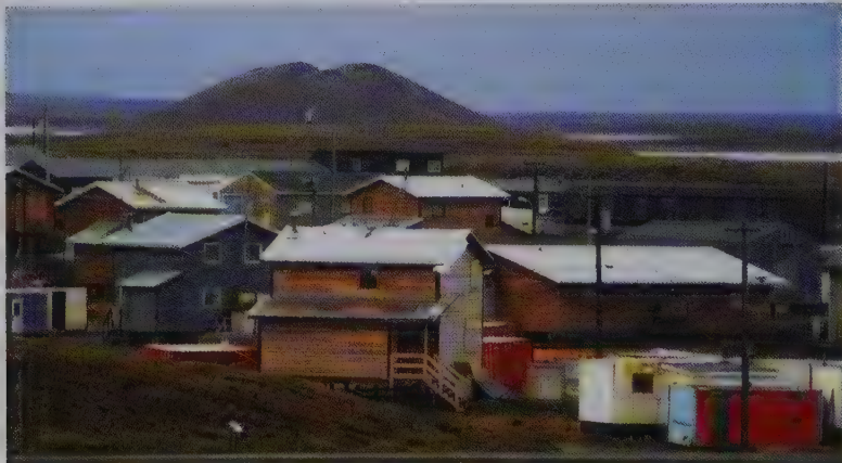
Colour Plate 13 Pingo beside Tuktoyaktuk, an Inuit village on the Mackenzie delta on the Arctic coast of North West Territories, Canada. The houses all stand on piles bored into the permafrost.
