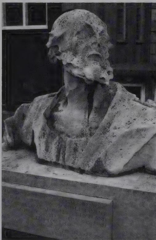
Plate 5.2 A bust of Saint Andrew, removed from St Paul's Cathedral because of accelerated decay.
