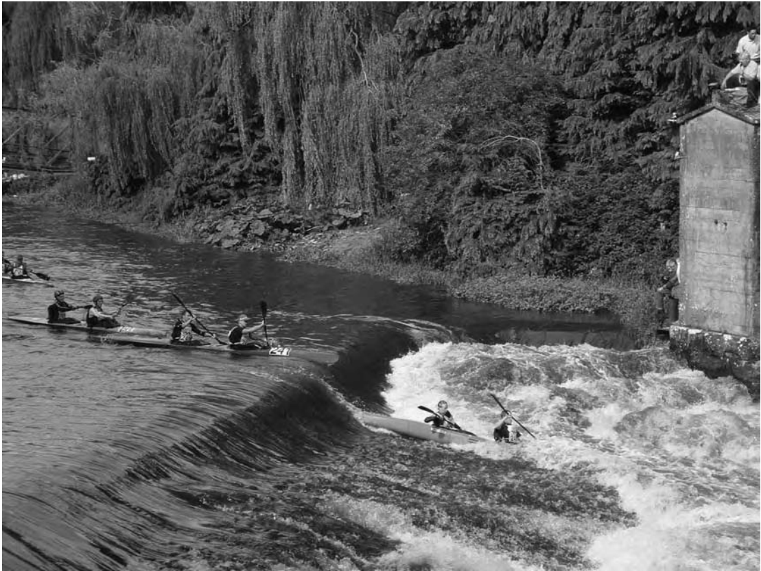
Plate 6.1 Hydraulic drop and hydraulic jump at a weir on the River Liffey, Country Kildare, Irish Republic. Photograph by Jeanne Meldon.
