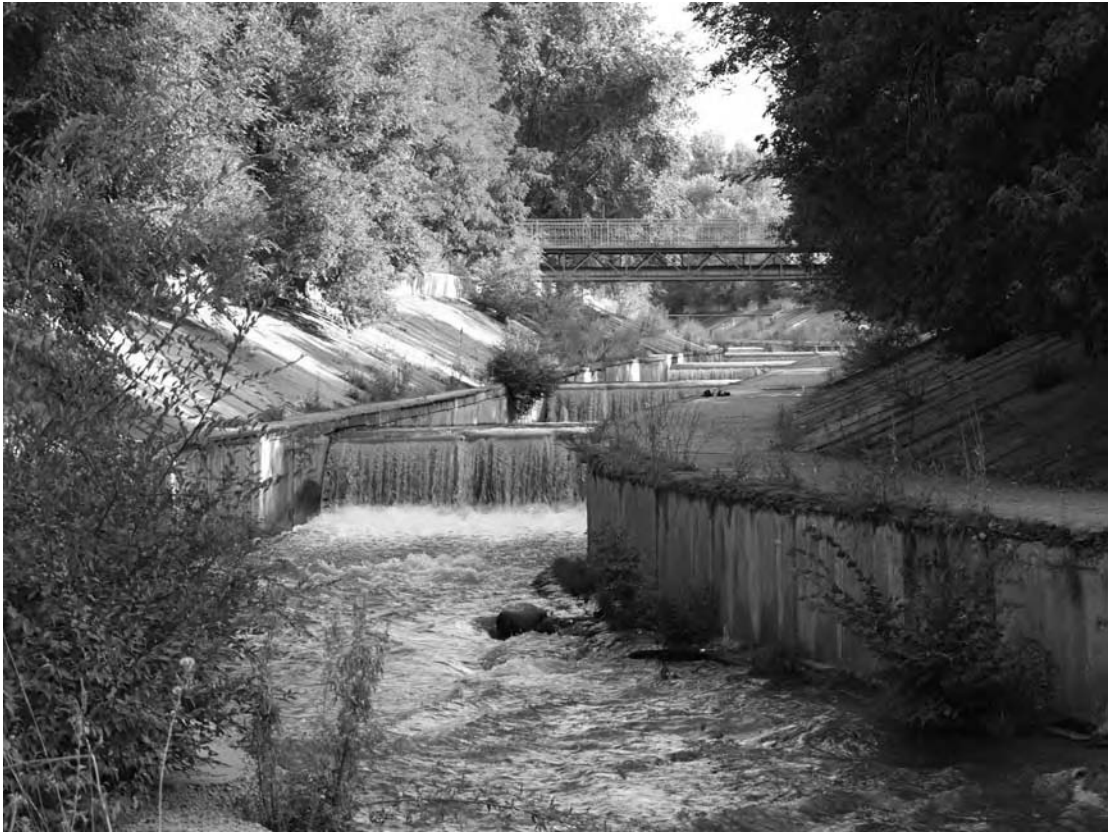
Plate 10.1 A steep, concrete-lined channel with grade control structures (weirs), Almaty, Kazakhstan.
