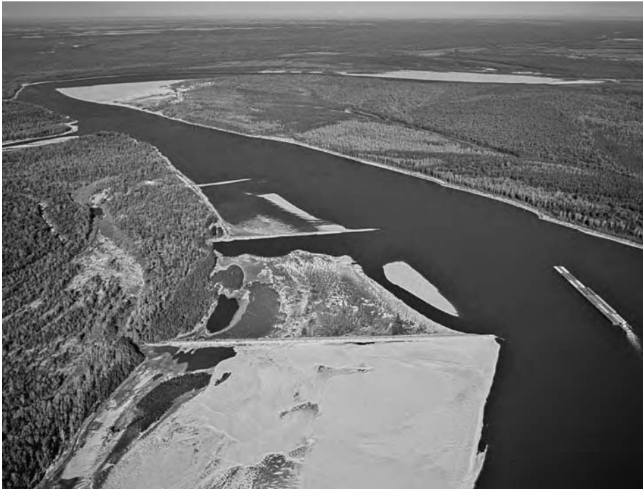
Plate 10.2 Spur dykes on the lower Mississippi, near Rosedale, Mississippi, United States. These encourage deposition, narrowing the channel and increasing flow velocity. In this way the depth of the navigation channel can be maintained. Photograph by Airphoto, Jim Wark.
