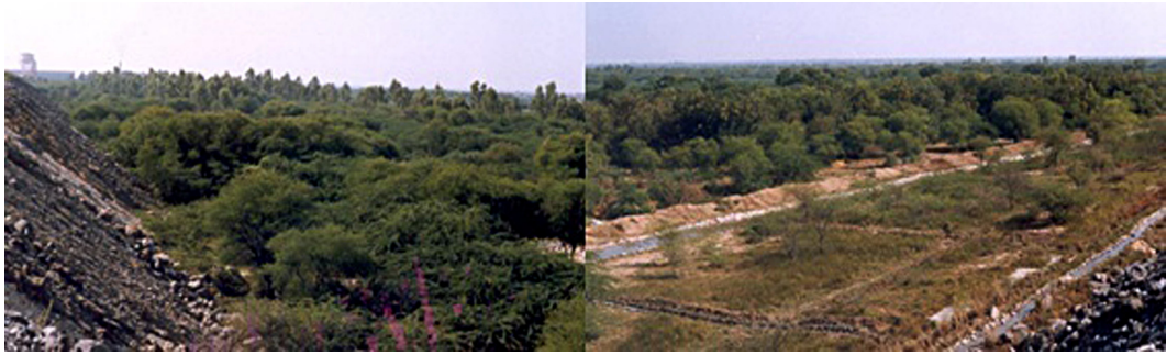
FIGURE A.14 (Left) Garland drains to prevent flooding of mine and contamination of natural water courses. (Right) Plantation near waste rock dump area. Source: Photo courtesy by Gandhi.
