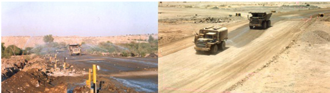
FIGURE A.13 Sprinkling of water (by sprinklers and water tank) on the haulage way, to suppress the dust in Rampura-Agucha mine complex. Source: Photo courtesy by Gandhi.
