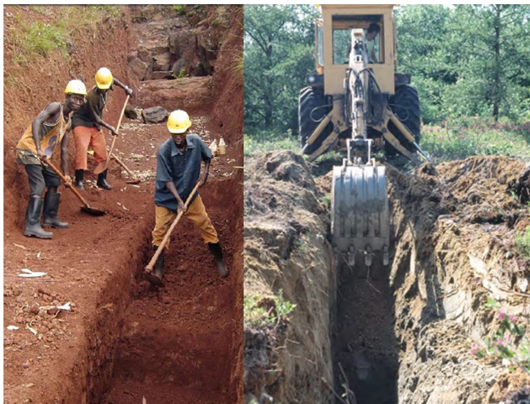
FIGURE 3.3 Trenching in gold prospects in West Africa. Courtesy: BURKINA 95.
