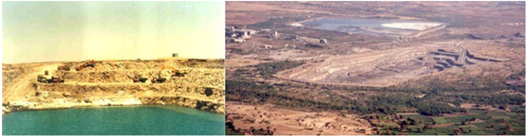
FIGURE A.8 Left: Pilot-pit operation in Rampura-Agucha in December 1988. Right: Aerial view of Rampura-Agucha open-pit mine, as in October 1999. Source: Photo courtesy by Gandhi.
