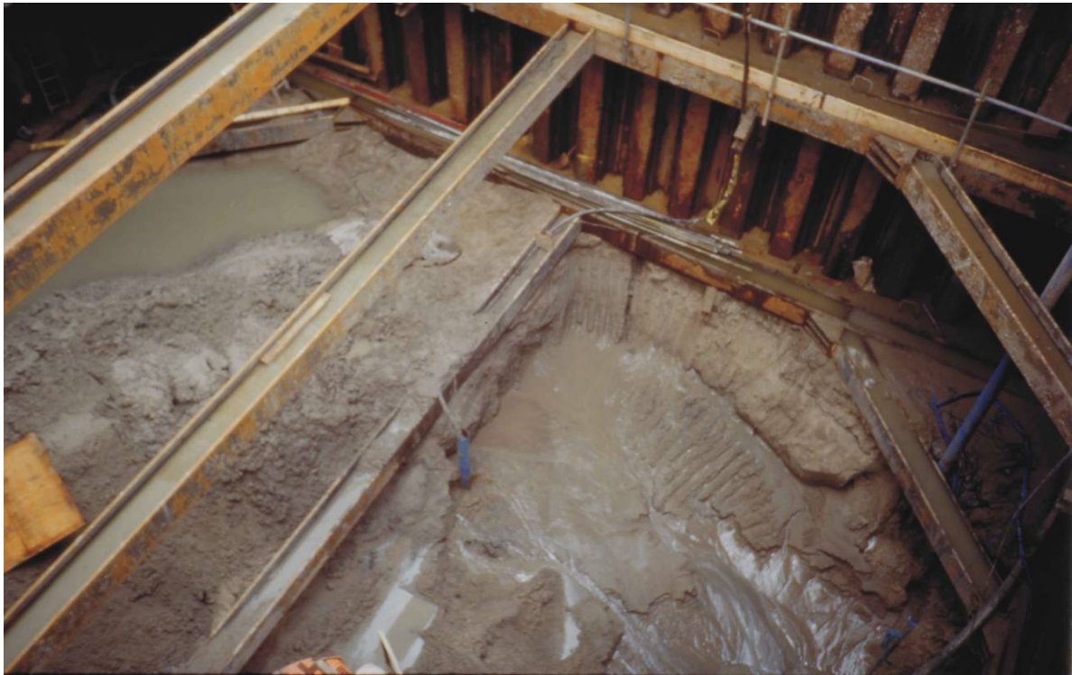
Figure 7.17. Excavation for the Jubilee Line Extension in Bermondsey, south London, showing grey sands infilling a channel that cut down into the Upper Mottled Clay Reading Formation. (Copyright Jackie Skipper).
