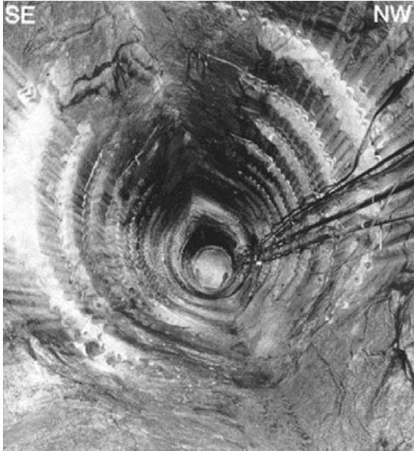
Fig. 7.4. Breakout in a circular tunnel with a radius of R = 1.75 m in the Underground Research Laboratory, Canada. The maximum breakout occurred in the minimum stress direction and the maximum hole radius is 1.3R . The in-situ stresses are \sigma_3 = 14 MPa and \sigma_1 = 55 MPa (Martino and Chandler 2004 with permission of Elsevier).
