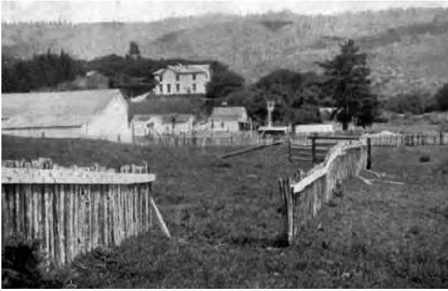
Earthquakes and Crustal Deformation, Figure 3 Picture taken in Marin County shows a fence that was offset about 10 ft along the trace of the San Andreas fault by the 1906 earthquake (Photo attributed to G.K. Gilbert; http://americahurrah.com/USGS/26.htm ).
