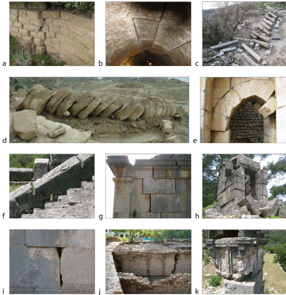
Archaeoseismology, Figure 1 Examples of deformations and damages which possibly are earthquake effects: (a) Horizontally deformed wall of a crusader fortress build on top of the Dead Sea Transform Fault in the Jordan Valley; (b) deformed vault of a Roman sewer in Cologne, Germany; (c) toppled columns of a Byzantine church in Sussita located above the Sea of Galilee; (d) toppled column of the great palace in Patra, Jordan; (e) moved block in an arch of the Nimrod fortress in the Golan Heights; (f) shifted blocks of an analemma of a Roman theatre in Pinara, SW Turkey; (g) moved blocks of a corner wall of a Roman monument in Patara, SW Turkey; (h) shifted blocks of a Roman grave house in Pinara, SW Turkey; (i) spall of block corners, same object as in (g); (j) broken and horizontally displaced fortification wall of the Roman Tolbiacum (Zülpich, Germany); (k) rotated Lycien sarcophagus in Pinara, SW Turkey.
