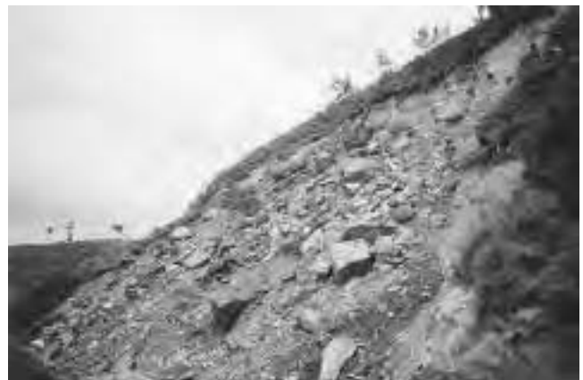
Roadside slump in Wutai Shan, China. A rain-soaked oversteepened slope failed, causing soil and rock to slump downhill, blocking the road. Note the tilted telephone poles on the slumped area. (Photo by Timothy Kusky)
