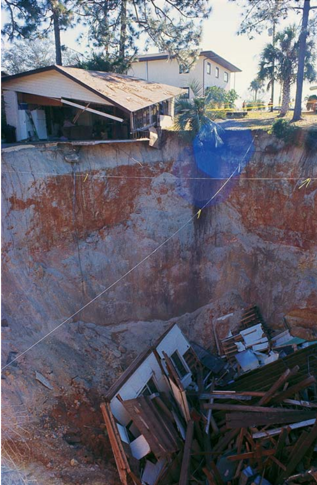
FIGURE 3 The remnants of a home engulfed as a large cover-collapse sinkhole developed over several hours, Keystone Heights, Florida (east of Gainesville). The occupants were able to evacuate safely, although their Christmas tree and presents were lost. The surficial sediment is clayey sand, which spans the upward eroding subsurface void allowing it to grow to a significant size before it collapsed. The limestone at this location is approximately 100 feet below the land surface. (Photograph courtesy of Barry F. Beck.)
