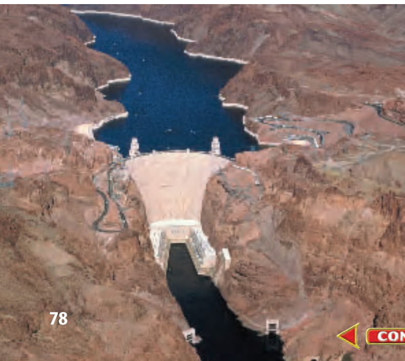
Figure 13 Hydroelectric power is important in many regions of the United States. Hoover Dam was built on the Colorado River to supply electricity for a large area.
