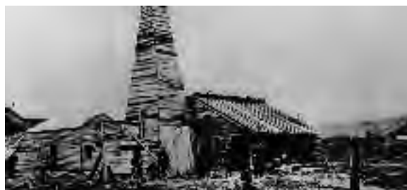
The Titusville, Pennsylvania, oil well drilled by Edwin Drake. This photo was taken in 1864.
