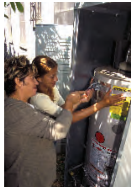
Figure 22 Sturdy metal straps on this gas water heater help reduce the danger of fires from broken gas lines during an earthquake.
