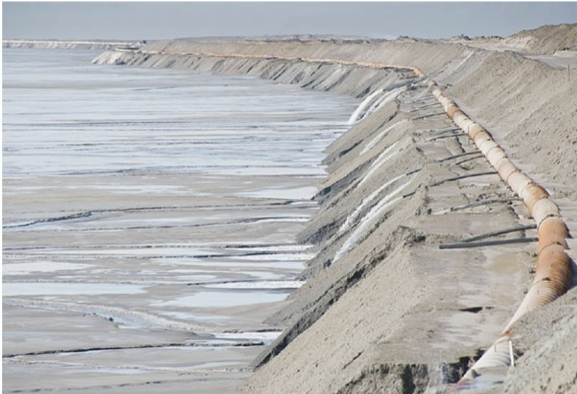
Figure 16.10 An active tailings pond in the vicinity of the Bingham Canyon Mine. (Photograph courtesy of Rio Tinto, Kennecott Utah Copper.)
