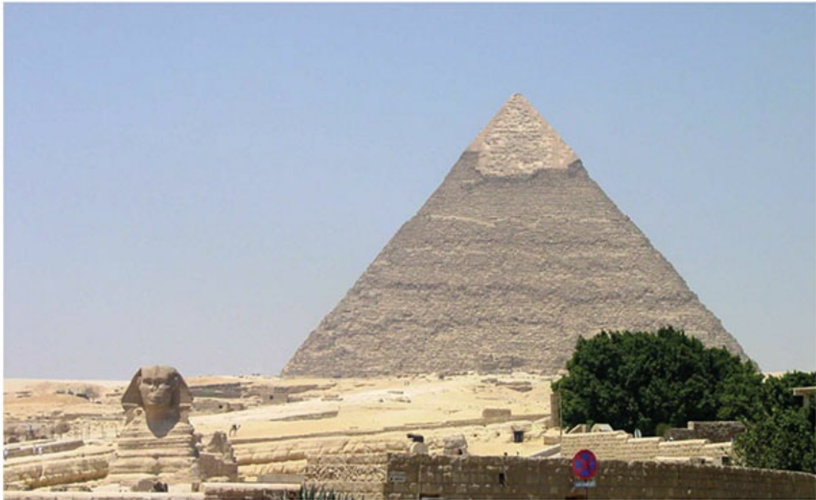
Figure 12.27 The pyramid of Khafre (Chephren) at Giza, Egypt, is built from the local Middle Eocene Mokattam Formation, a nummulitic (foram) packstone, which forms the gently dipping layers in the foreground. The Sphinx is carved from this same limestone. (Photograph courtesy of Vivian Rigg.)
