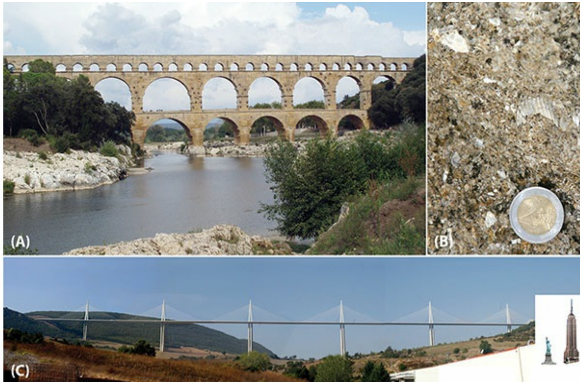
Figure 16.3 (A) The Pont du Gard, a Roman aqueduct, brought water to nearby Nimes in southern France. (B) Limestone used in the construction of the Pont du Gard. (C) Bridge at Millau, France, is made of concrete and steel. Inset shows the heights of the Statue of Liberty and the Empire State Building, New York City, relative to the Millau Bridge.
