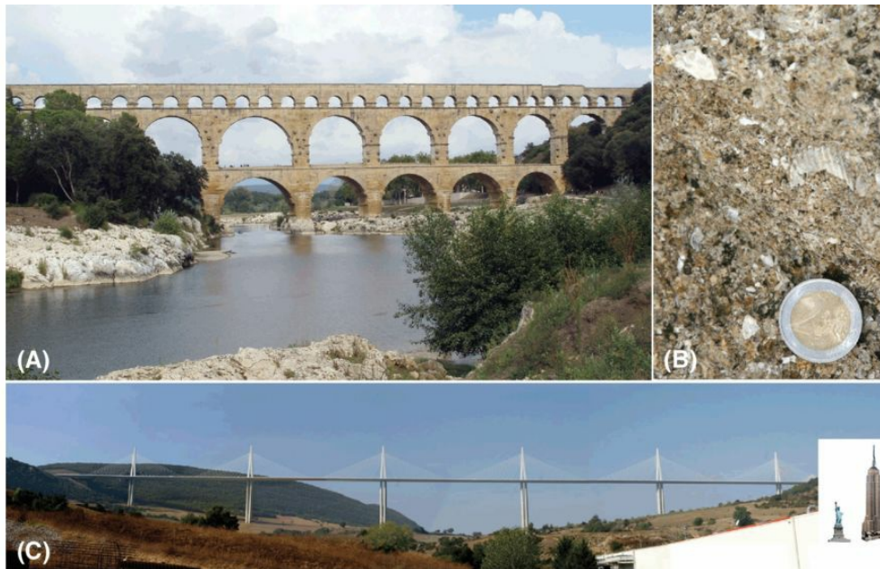
Figure 17.3 (A) The Pont du Gard, a Roman aqueduct, brought water to nearby Nimes in southern France. (B) Limestone used in the construction of the Pont du Gard. (C) Bridge at Millau, France, is made of concrete and steel. Inset shows the heights of the Statue of Liberty and the Empire State
