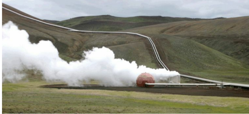
Figure 17.16 Geothermal well head (red geodesic dome) with steam rising from the adjoining relief valve and pipes feeding the superheated steam into the power-generating plant at the Krafla Volcano, Iceland.
