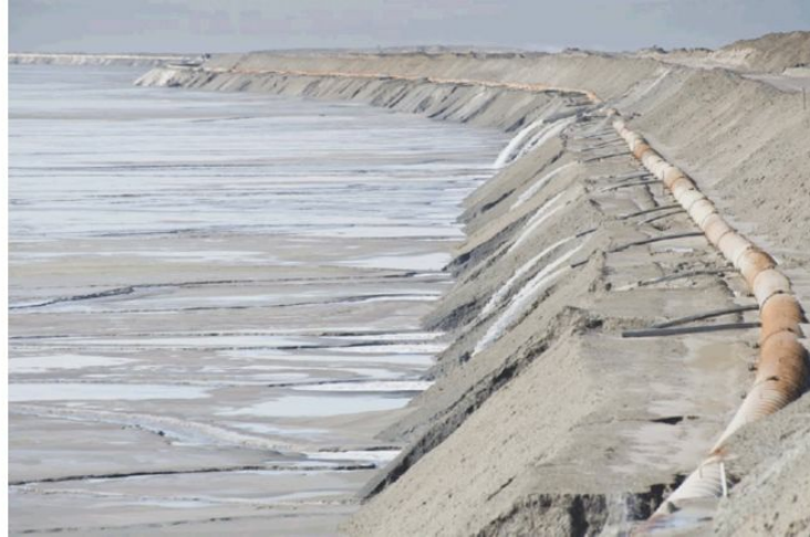
Figure 17.10 An active tailings pond in the vicinity of the Bingham Canyon Mine.
