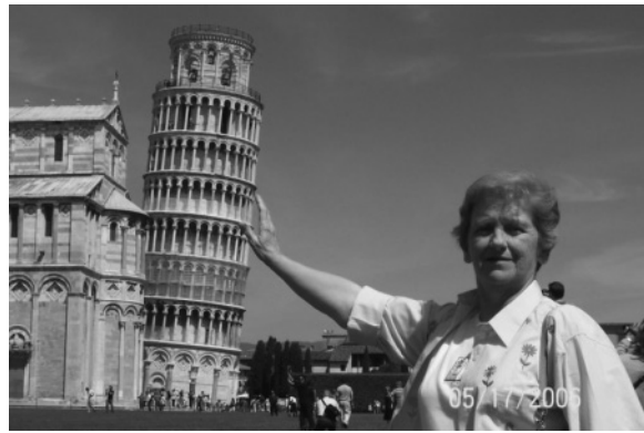
Figure 12.25 Italy's famed Leaning Tower of Pisa, which was constructed on compressible, clay-rich soil. As a result of differential consolidation, the tower requires additional reinforcement (here supplied by Maureen Crowe) to maintain its equilibrium. (Photo courtesy of Tony Crowe.) (For color version, see Plate 12.25, between pp. 248 and 249.)
