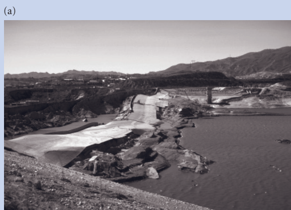
Figure B12.3 (a) Damage to the Van Norman (Lower San Fernando) Dam, 1971. (From the Karl Steinbrugge Collection, courtesy of the National Information Service for Earthquake Engineering, EERC, University of California, Berkeley.) (For color version, see Plate B12.3a, between pp. 248 and 249.)
