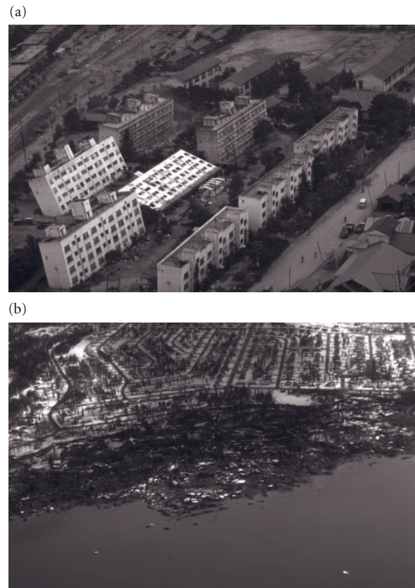
Figure 12.23 (a) Collapsed apartment buildings in Nigata, Japan, after the 1964 earthquake. (b) Neighborhood in Anchorage, Alaska, destroyed when the ground slumped, carrying structures more than 1 km, after sand lenses became liquefied during another 1964 earthquake. (From the Karl Steinbrugge Collection, courtesy of the National Information Service for Earthquake Engineering, EERC, University of California, Berkeley.) (For color version, see Plate 12.23, between pp. 248 and 249.)
