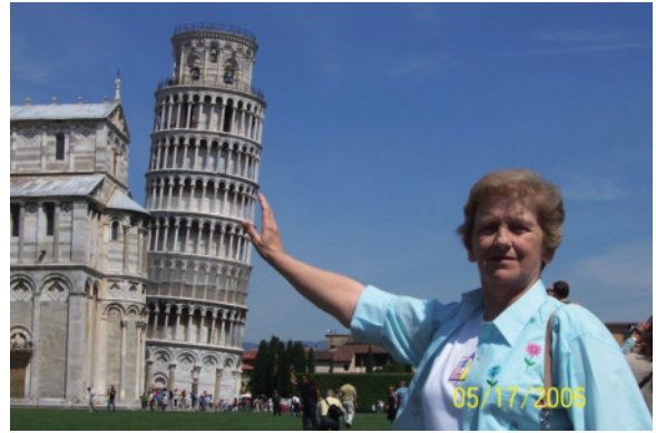
Plate 12.25 Italy's famed Leaning Tower of Pisa, which was constructed on compressible, clay-rich soil. As a result of differential consolidation, the tower requires additional reinforcement (here supplied by Maureen Crowe) to maintain its equilibrium. (Photo courtesy of Tony Crowe.)
