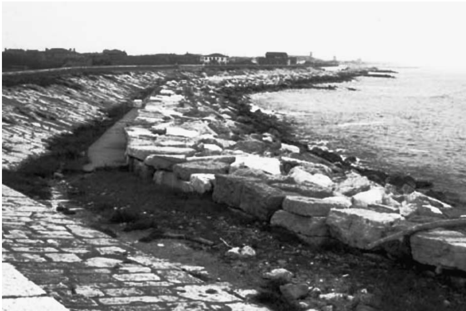
Figure 14.3 An artificial coastline formed after a sea wall and groynes failed to retain the beach at Litorale di Pellestrina, near Venice (location shown in Figure 11.10) on the coast of Italy, and limestone blocks were dumped on the shore
