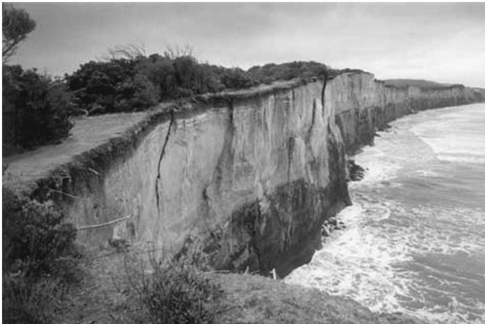
Figure 4.7 Cracks in the mudrock cliff at Demons Bluff, Victoria, Australia, which recedes as masses of rock fall from the cliff face
