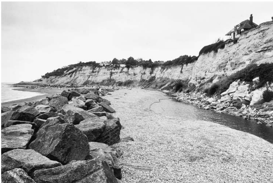
Figure 14.2 Desperate remedies. A boulder bank has been built on the shingle beach at Fairlight Cove, Sussex, in an attempt to exclude wave action and so halt the cliff recession which has destroyed several houses. As sea level rises, this kind of problem will become more widespread
