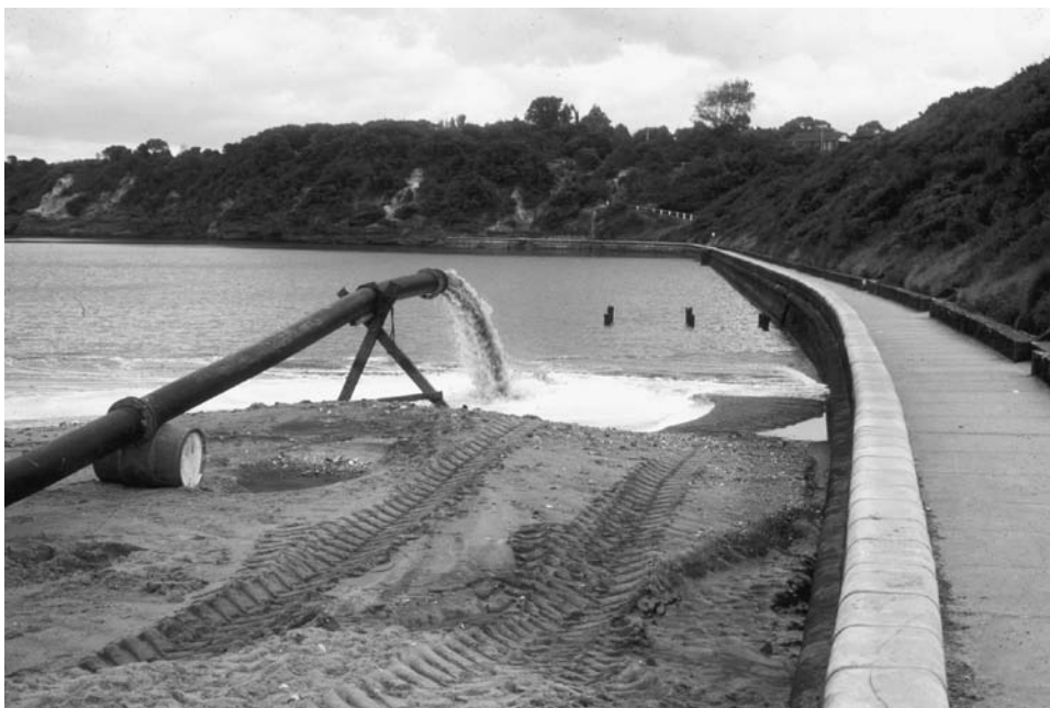
Figure 7.8 Beach nourishment in progress at Mentone, Port Phillip Bay, Australia
