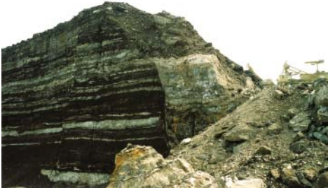
Figure 2.38 Highwall termination due to faulting in Palaeogene–Neogene brown coal opencast mine in Bosnia-Herzegovina. Source: Photograph by courtesy of Dargo Associates Ltd.
