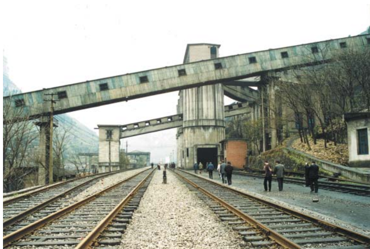
Figure 13.2 Coal silos for loading coal directly to trains, the PRC. Source: Photograph by courtesy of Dargo Associates Ltd.
