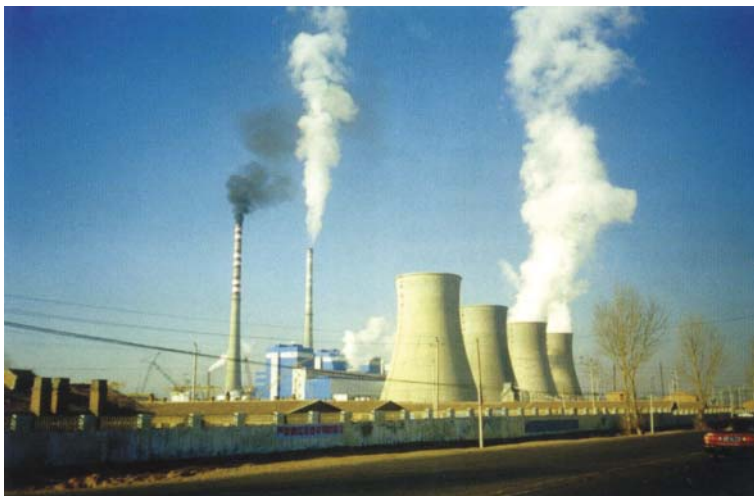
Figure 12.13 Modern coal-fired power station, Inner Mongolia, PRC. Source: Photograph courtesy of Dargo Associates Ltd.
