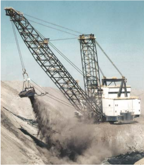
Figure 10.15 Dragline removing overburden in open-pit mine, USA.
