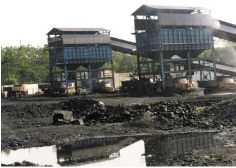
Figure 13.6 Automatic loading of trucks from overhead bins, Orissa State, India. Source: Photograph by courtesy of Dargo Associates Ltd.
