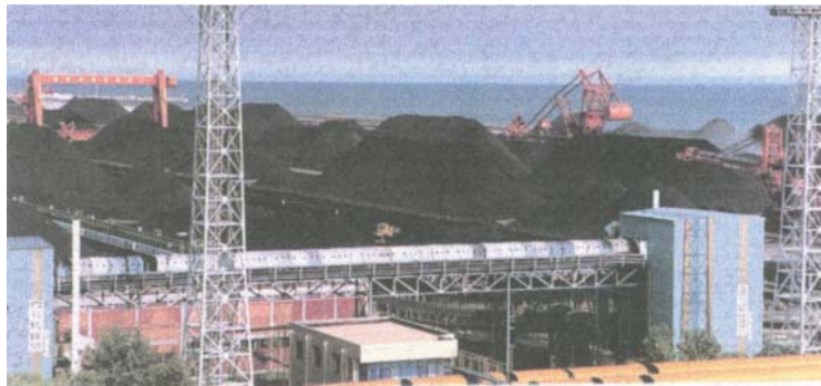
Figure 13.3 Modern coal stockyard at port of Qinhuangdao, PRC. Source: Photograph by courtesy of Dargo Associates Ltd.
