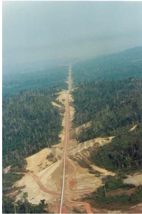
Figure 13.4 Overland conveyor, 14 km in length, from Kaltim Prima Coalmine to the port of Tanjung Bara, East Kalimantan, Indonesia. Source: Photograph by courtesy of Dargo Associates Ltd.
