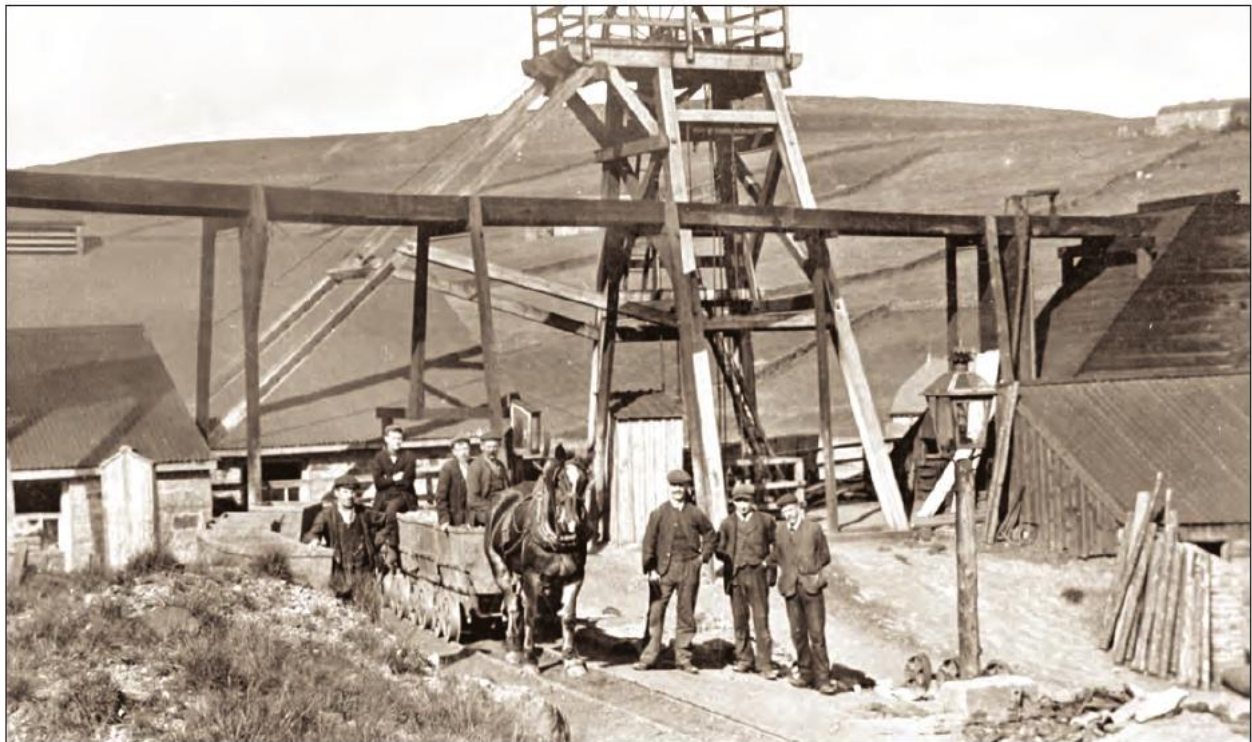
Headframe of the Boltsburn mine, ca. 1910. Beamish Museum photo archives.
