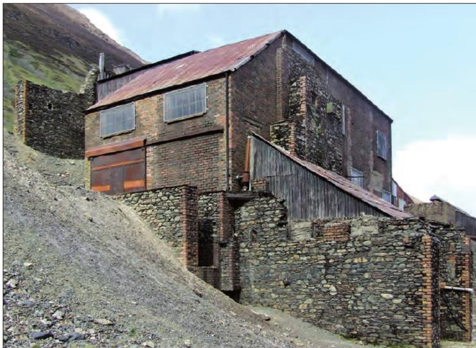
Surface structures at the Force Crag mine. Gordon Akitt photo.
