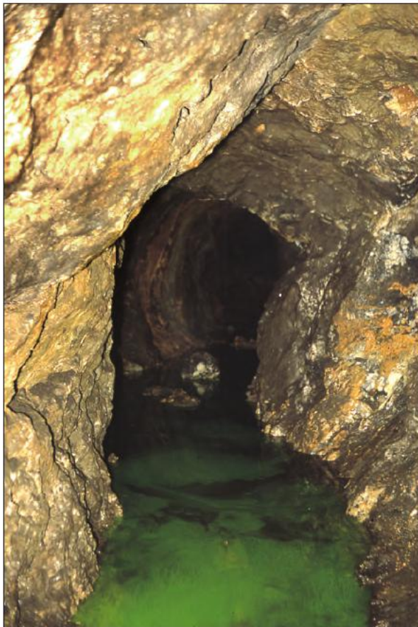
Interior of an adit leading into the Dry Gill mine.
