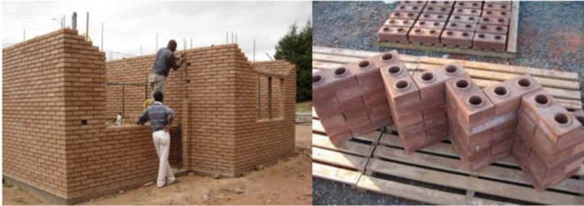
Figure 1. Soil cementer construction
