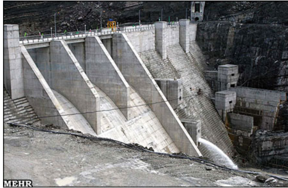
Fig. 1.28 RCC Jagin Dam in Iran
