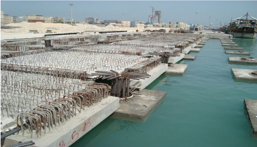
Fig. 4.23 Bushehr port complex under construction with silica fume concrete
