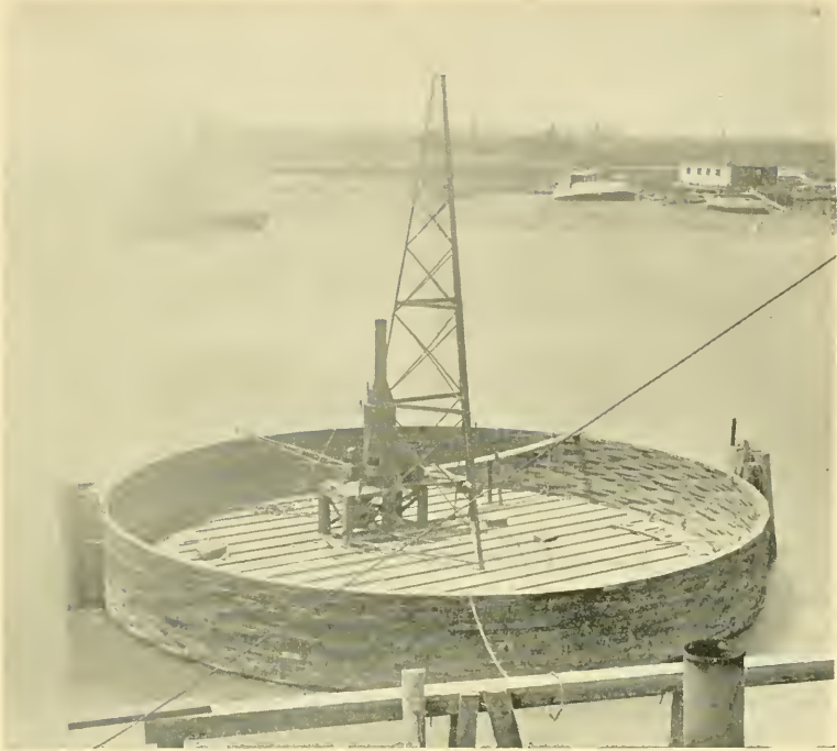
EARLY STAGE IN CONSTRUCTION OF WEBSTER-STREET DRAW-BRIDGE PIER.
