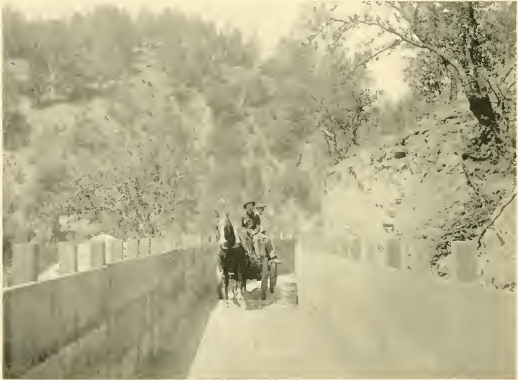
FLUME TO CARRY 600 MINER'S INCHES OF WATER FROM THE STANISLAUS RIVER TO THE 120-STAMP MILL AT THE MELONES MINE.
