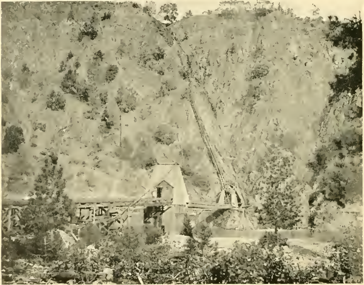
SUSPENSION BRIDGE ACROSS TRINITY RIVER, AT JUNCTION CITY.
