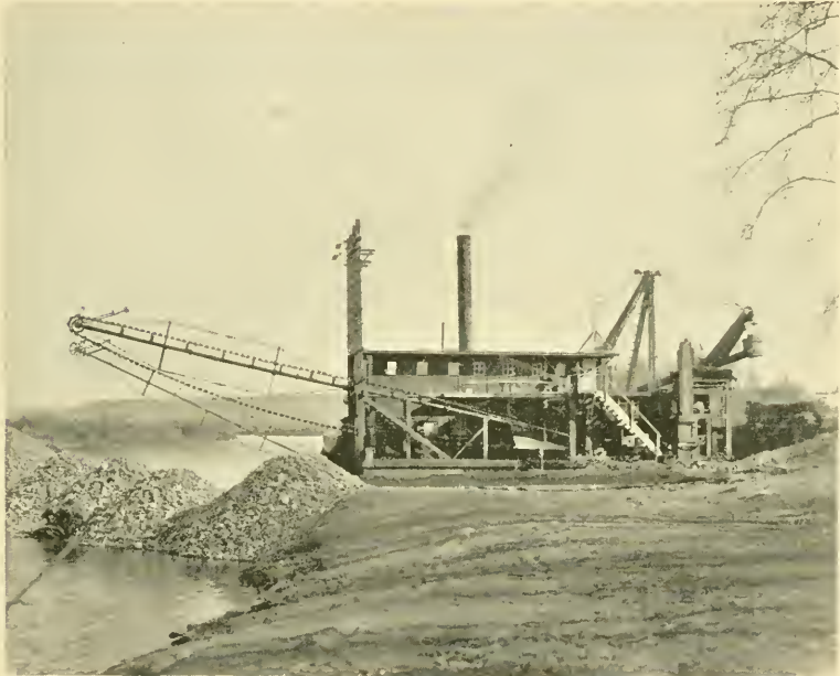
DREDGE OPERATING ON FEATHER RIVER.
