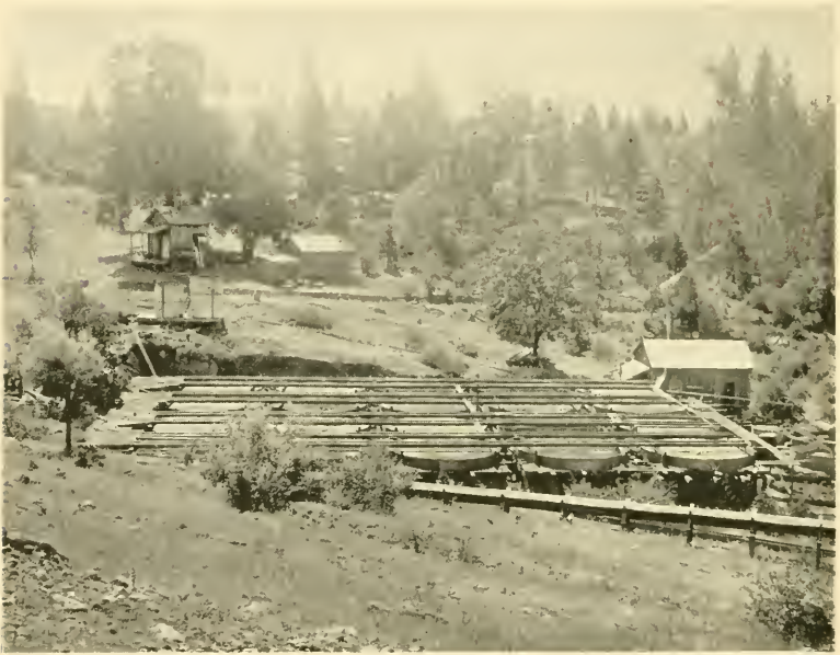
CYANIDE PLANT, TAYLOR MINE.
