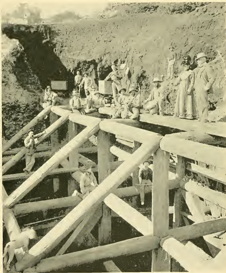
OPEN STOPE IN THE ALMADEN QUICKSILVER MINE.
