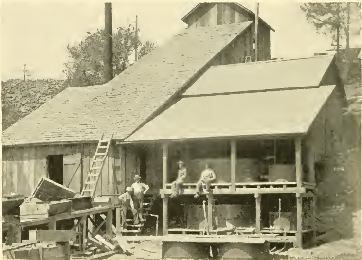
SMALL TEN-TON EXPERIMENTAL CYANIDE PLANT AT THE MELONES MINE.
