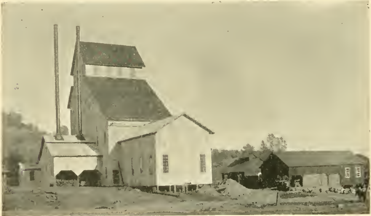
COMPLETED HOISTING WORKS AT THE ONEIDA MINE.
