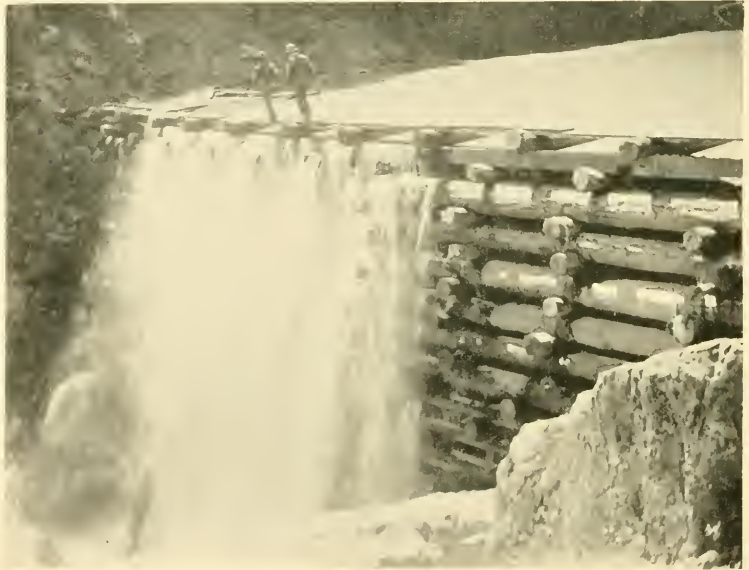
DEBRIS-RESTRAINING DAM BELOW THE RED DOG HYDRAULIC MINE, NEVADA COUNTY.
