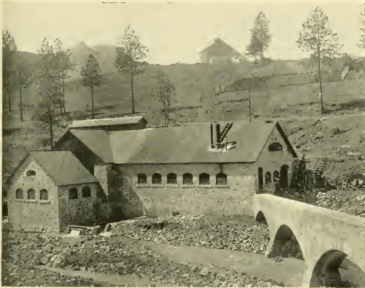
COMPRESSED AIR POWER-HOUSE. NORTH STAR MINE, GRASS VALLEY.
