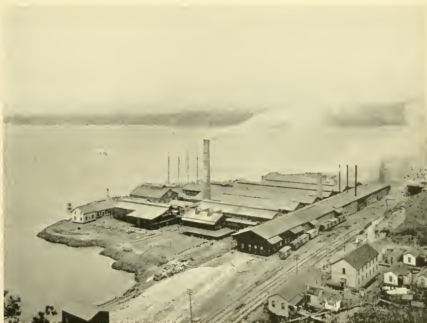
Selby Smelting and Lead Company's Works at Vallejo Junction.
