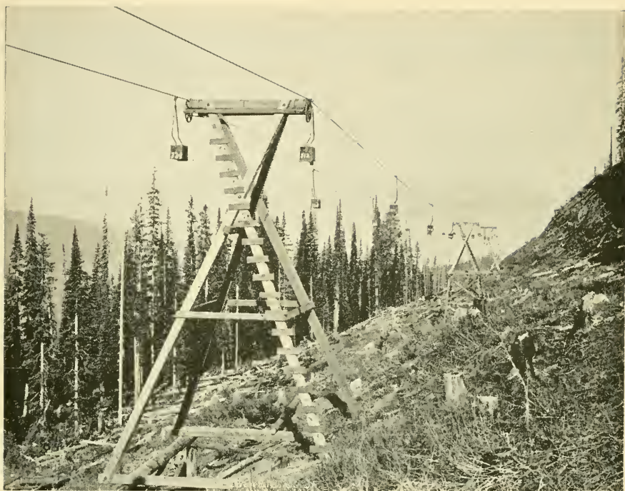
View of Towers on Ropeway at Hall Mines, Nelson, B. C.
