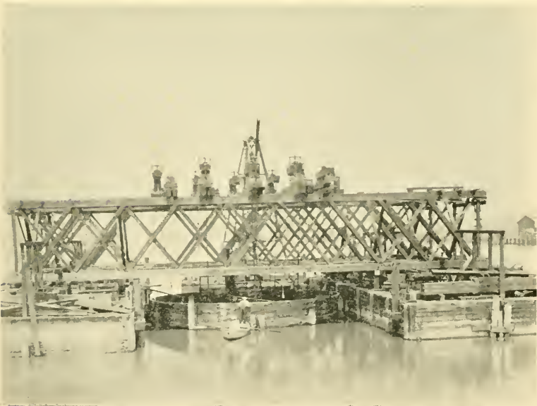
PLACING THE TRUSS OVER THE CENTER PIER.
