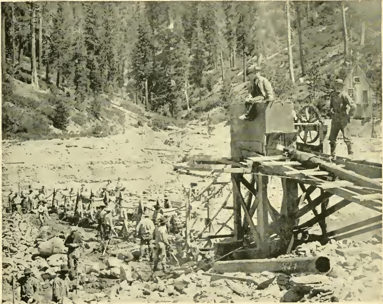
SHOWING THE INTERESTING METHOD OF OPERATING THE CONTINUOUS-LINK CARRIER AT THE ALTURAS MINE WITH AN IMPULSE WHEEL, THE USED WATER SUPPLYING THE PIPE.
