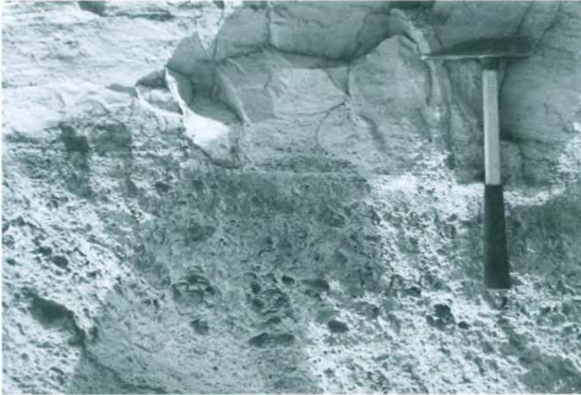
Fig. 9.18. Photograph of sequence boundary between Portland Limestone skeletal oolite and overlying Purbeck algal laminite (both late Jurassic), Isle of Portland, Dorset, England. Note biomoldic porosity beneath the contact. Adjacent to this locality fossil trees occur in growth position on the Portland oolite, testifying to the penecontemporaneous emergence and meteoric flushing of the oolite shoals.
