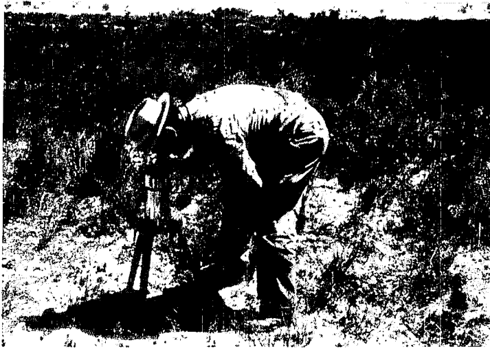
Figure 2.13. Reading a Worden gravimeter.
