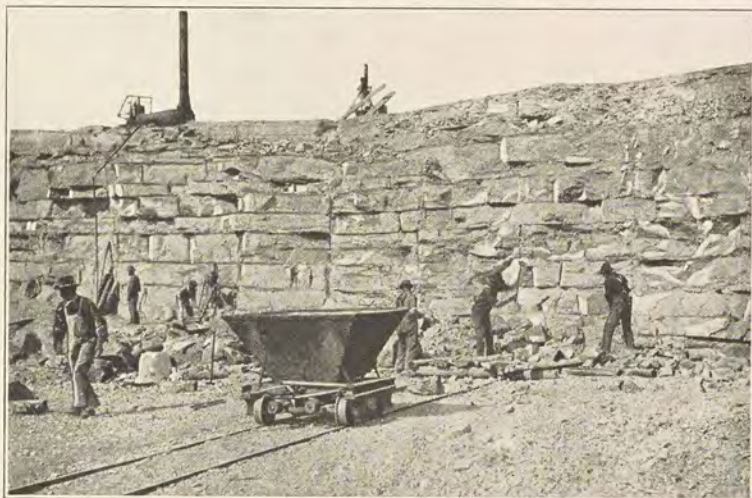
Fig. 64. Bluish hydraulic limestone of Devonian age, found near Milwaukee, Wisconsin
