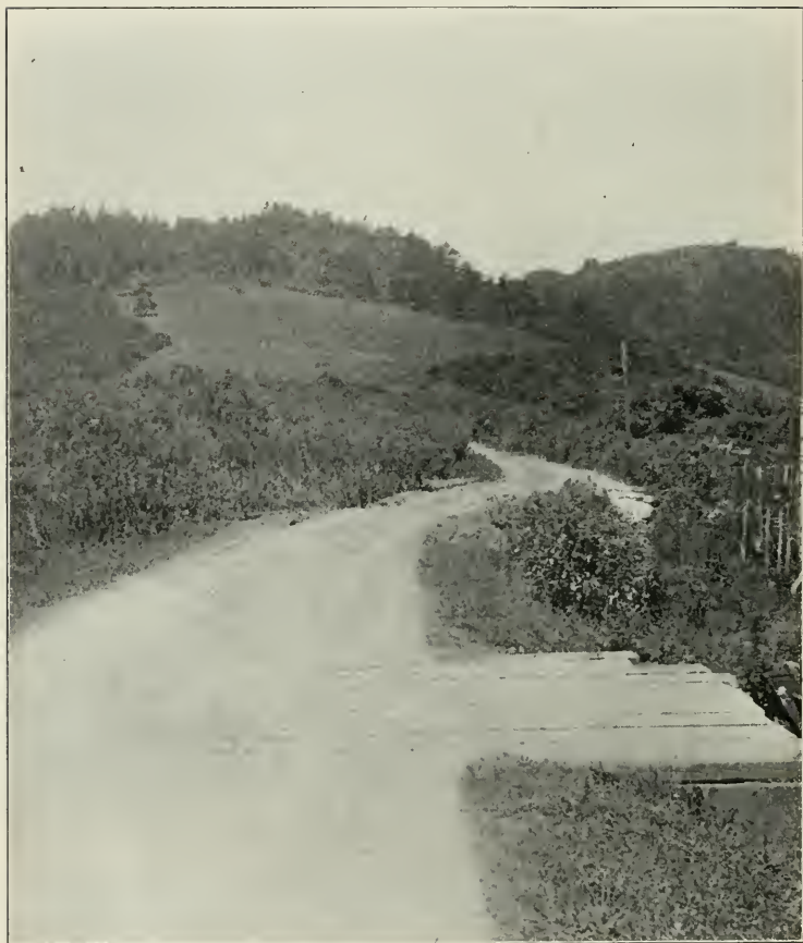
FIG. 9. — Horizontal shifting of the ground, San Francisco earthquake, 1906. Before the earthquake the road was straight. (Photograph by Sinclair)
