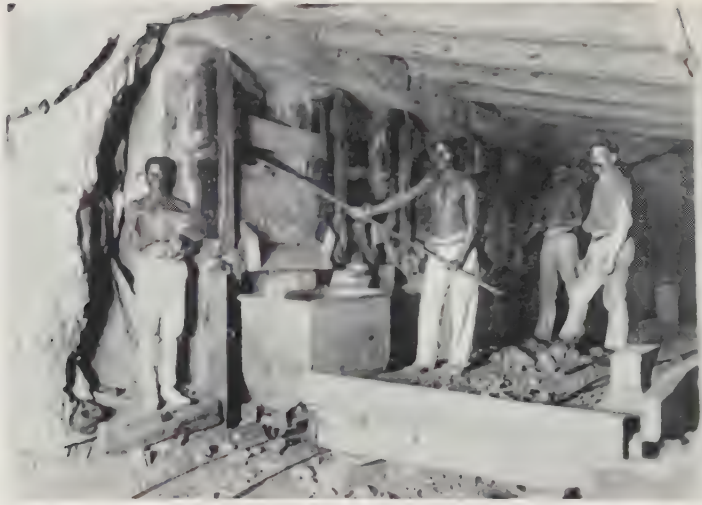
DeBeers Consolidated Mines, Ltd. LOADING AT AN ORE-PASS, KIMBERLEY
