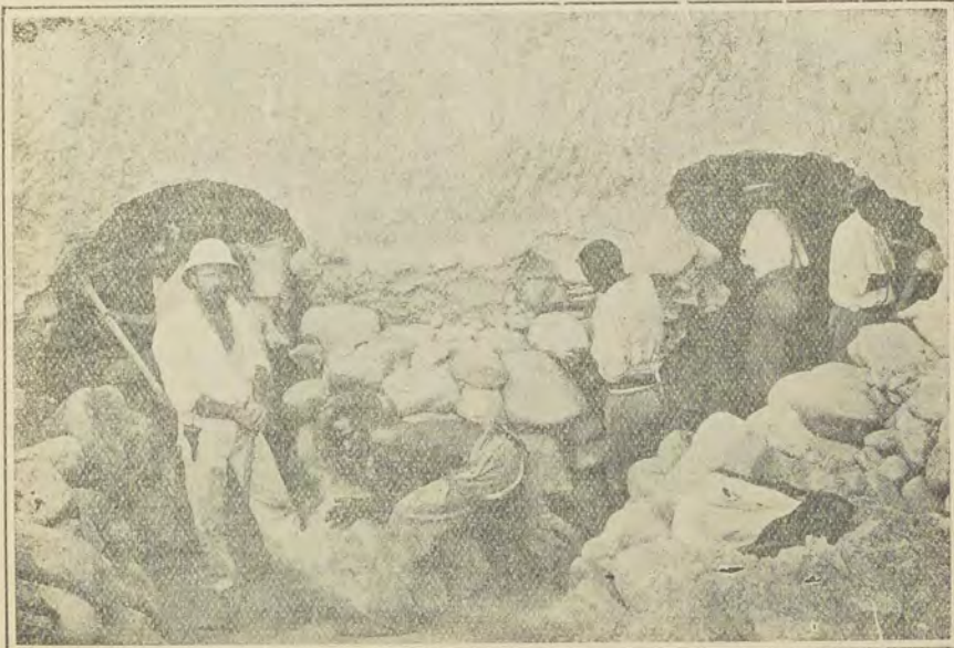
Working in River Bed, Sydney.
