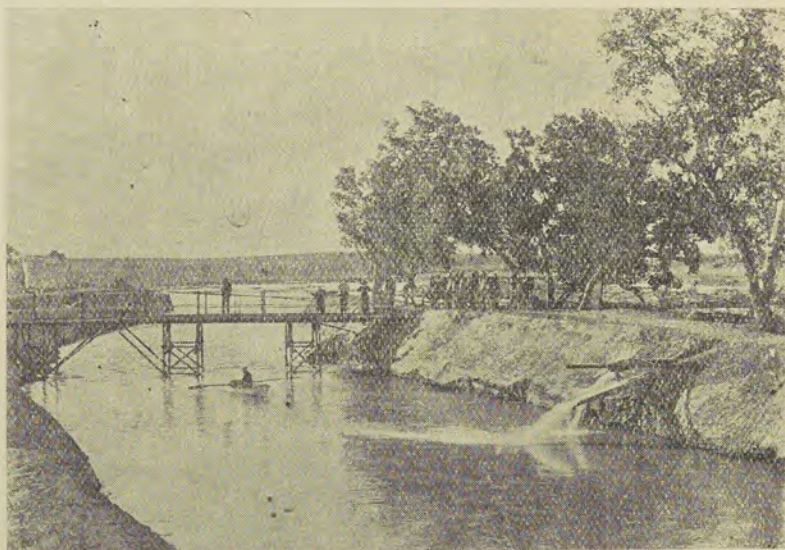
Outflow Channel and Bridge at Sydney Pont Pool Breakwater, 1910.
