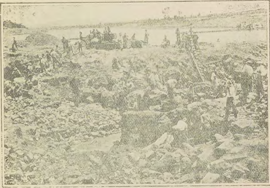
Work inside Breakwater, after water has been pumped out.
