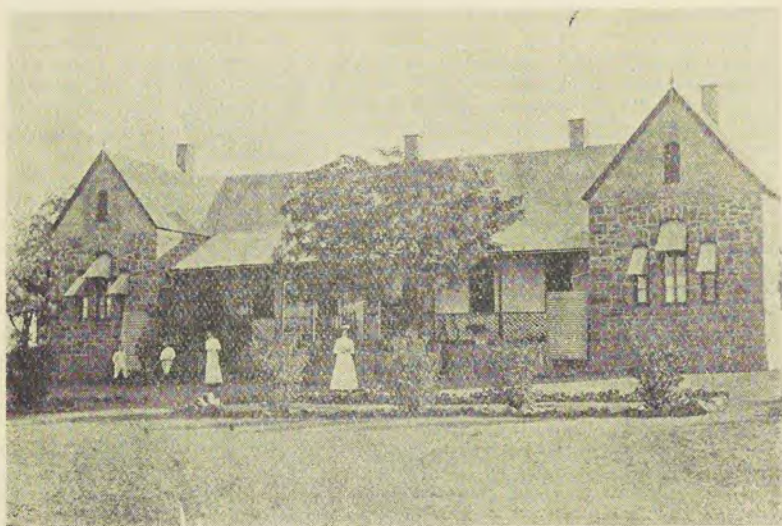
The Hospital, Barkly West.
