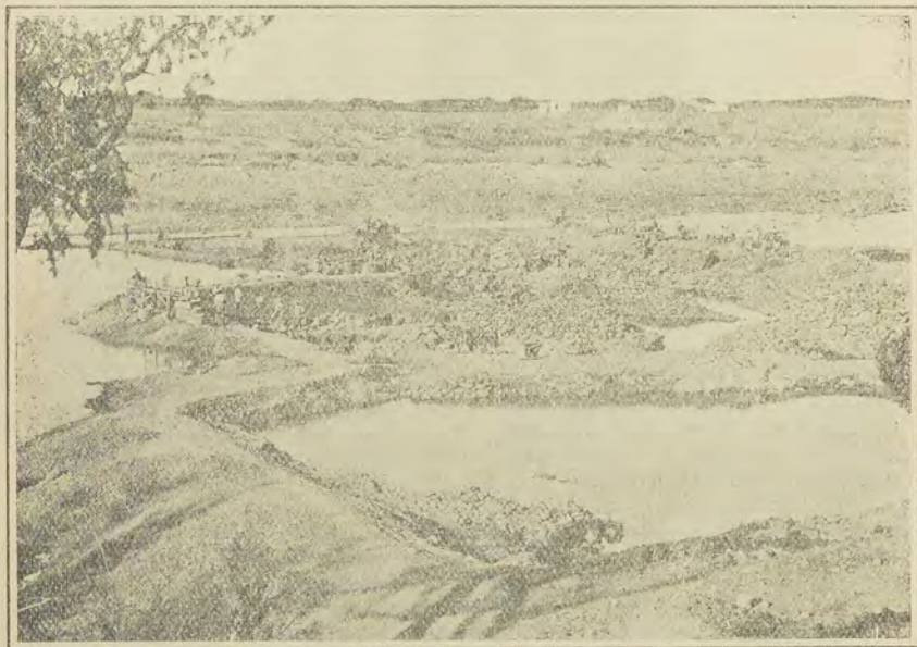
Delpoort's Hope Breakwater, water half pumped out.
