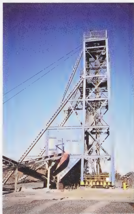
Figure 6. The headframe at Frank Smith mine in South Africa stands above the vertical access shaft to underground workings and controls the cable and cars moving in the shaft. (George E. Harlow.)
