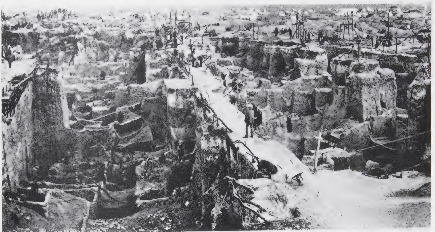
Figure 15. By 1872, as miners dug deeper, the walls that served as roadways between the claim pits at the Kimberley mine had started to collapse, making mining difficult and unsafe. The roadways, which ran north-south, were 15 feet wide, with 7.5 feet taken from the sides of each bordering claim ( 31 \times 31 feet), making the working surface of each claim 31 \times 23.5 feet. (From Williams, 1906; Jackie Beckett/courtesy of American Museum of Natural History.)
