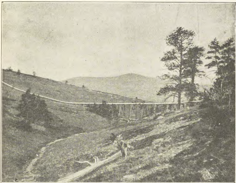
MONTANA SAPPHIRE MINING—WOODEN BRIDGE CARRYING PIPES TO THE WORKINGS.
