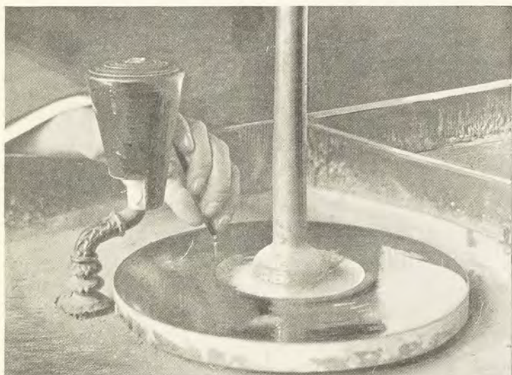
GEM HELD IN POSITION AGAINST THE WHEEL.
