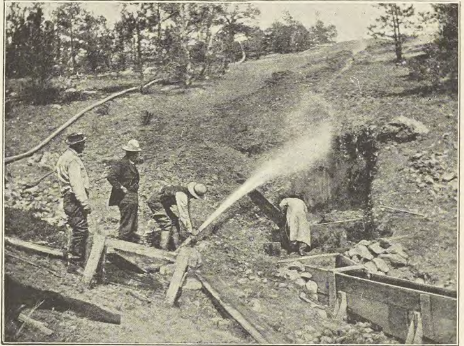
MONTANA SAPPHIRE MINING—A "NEW CUT."
