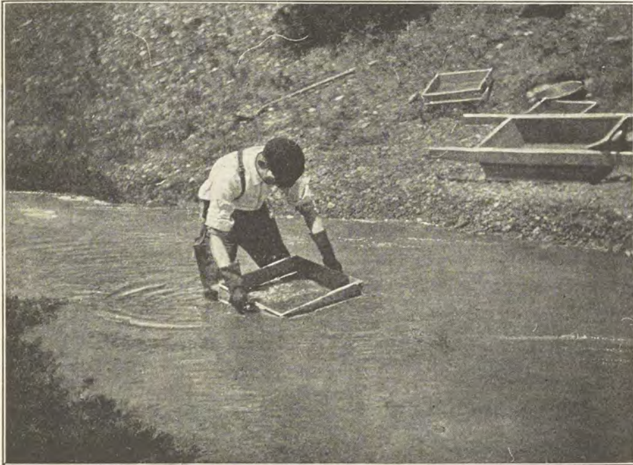
MONTANA SAPPHIRE MINING—WASHING THE GRAVEL AND DIVIDING IT INTO SIZES.
