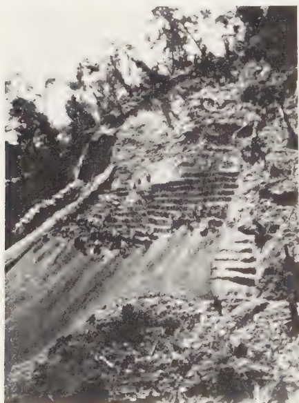
Figure 11.5 Views taken in the Chivor emerald mine about 1920, showing clearing of overburden (top photos) and development of the 'step' or 'benching' method to systematically excavate the emerald-bearing ground. From L. J. Canova, Chivor-Somondoco Emerald Mines of Colombia (New York, 1921)
