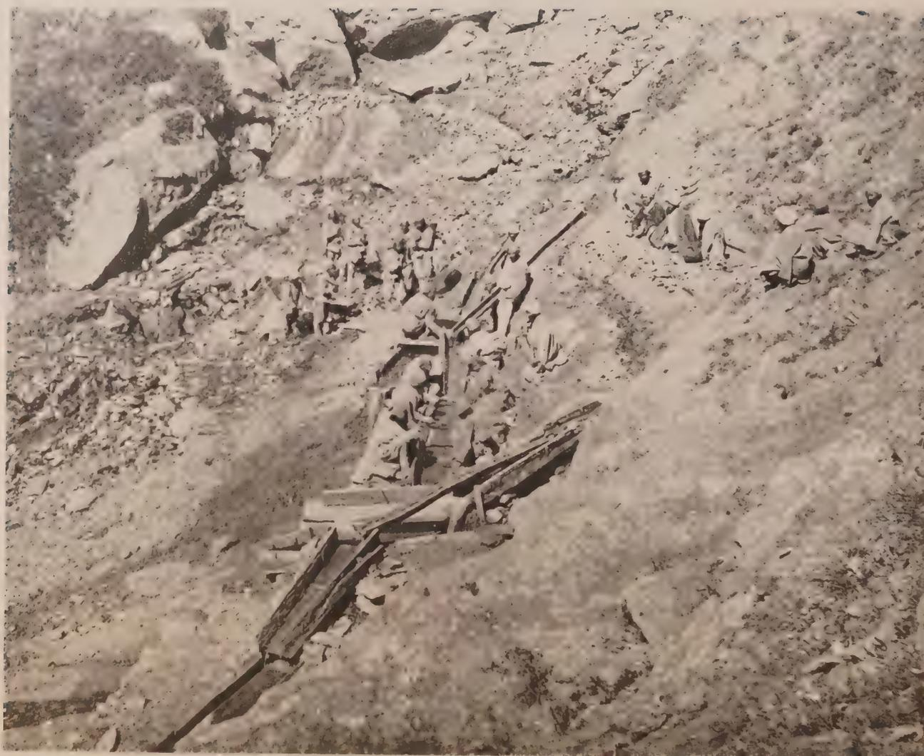
**Figure 12.65** The sapphire washing apparatus constructed by La Touche at the Kashmir mine. Taken in 1887–8, this is the earliest photo known of mining at this storied location. (From La Touche, 1890)
