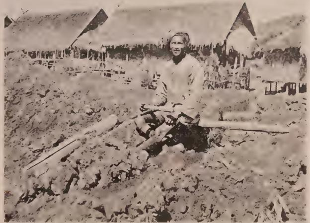
**Figure 12.39** A Burmese miner at Mogok dewatering an excavation using an ingenious bamboo pump. (From O'Connor, 1905)
