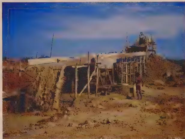
**Figure 12.132** Heavy media separation jig at Bo Rai, Trat Province, Thailand. Ruby-bearing earth is pumped into the jig where the heavy minerals, such as ruby, are separated from the lighter waste. (Photo: Wimon Manorotkul, ca. 1983)
