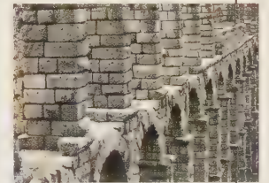
AQUEDUCT The aqueduct at Segovia, Spain, was built of Guadaramma granite during the reign of the Roman emperor Trajan (AD98–117). It is 728m (2,388ft) long and is still in use.
