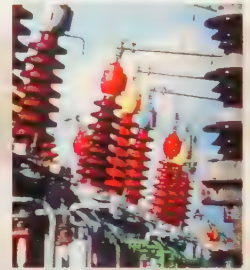
ELECTRICAL INSULATOR Ceramic electrical insulators use wollastonite due to its low conductivity.
