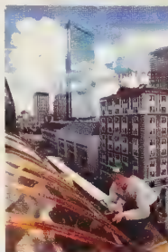
COPPER ROOFING Copper's malleability allows it to be used for curves.
