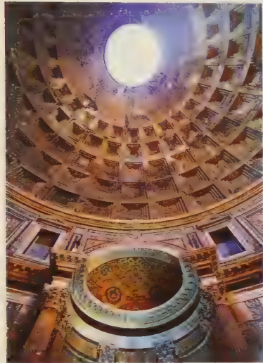
PANTHEON, ROME The dome of the Roman Pantheon was made from concrete mixed with pumice. This gave the mixture lightness and strength. Pumice is still used as a lightweight building aggregate.
