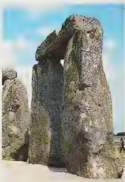
MORTISE AND TENON The lintels of the sandstone circle and trilithons are held on their uprights by mortise-and-tenon joints. The tenon can just be seen at the top of the far upright.
