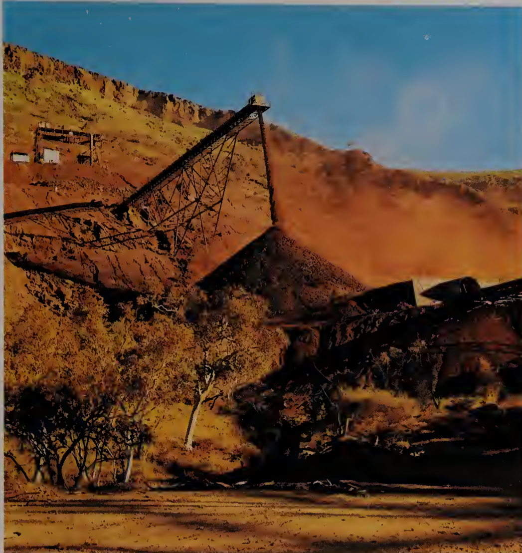
Above: Stockpiling crushed iron ore in the Hamersley Range of northwest Australia. It is estimated that this ore deposit contains 600 million tons of high grade hematite
