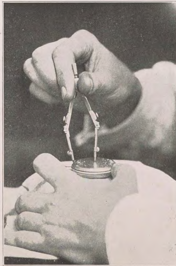
Finding Center of Watch Cases, Also Locket
