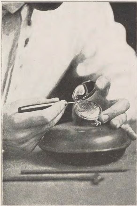
Correct Way of Taking Out Pin Before Engraving
