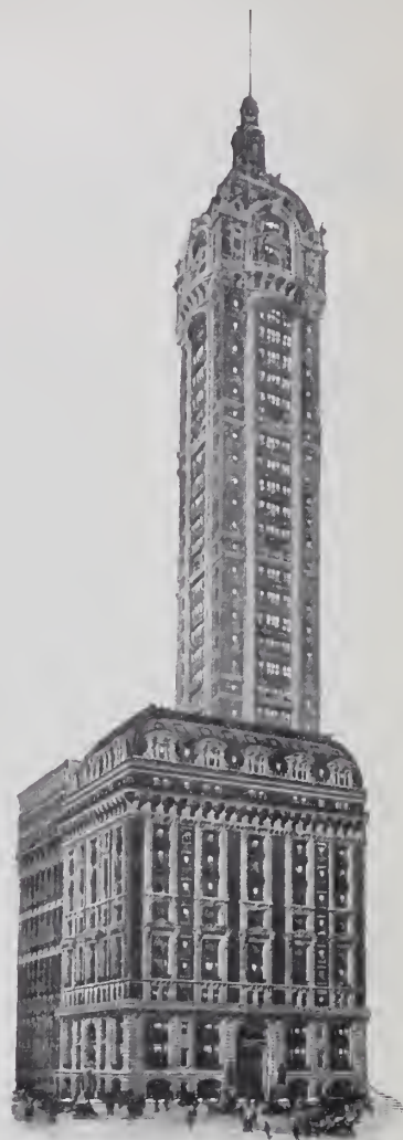
SINGER BUILDING, NEW YORK. Height, 612 ft. 1 in. Broadway, near Maiden Lane.
