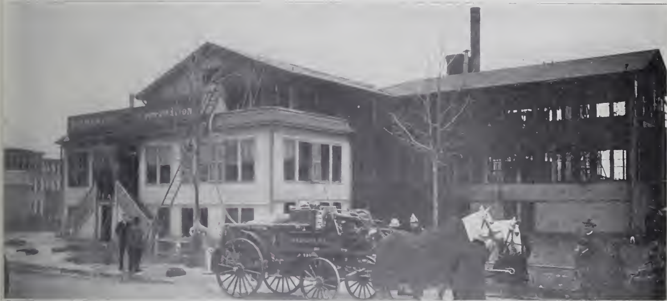
THE WILMARTH BUILDING AS IT LOOKED DIRECTLY AFTER THE FIRE.
