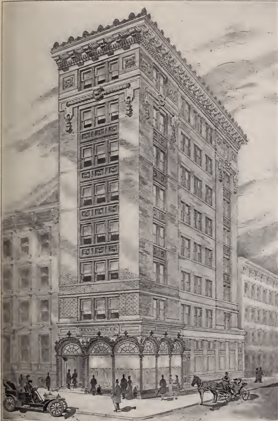
ALVIN BUILDING, IN COURSE OF CONSTRUCTION AT 35TH ST. AND FIFTH AVE., NEW YORK.
