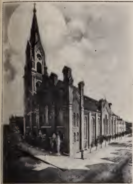
CLOCK IN TOWER OF ST. MICHAEL'S GERMAN CATHOLIC CHURCH.
