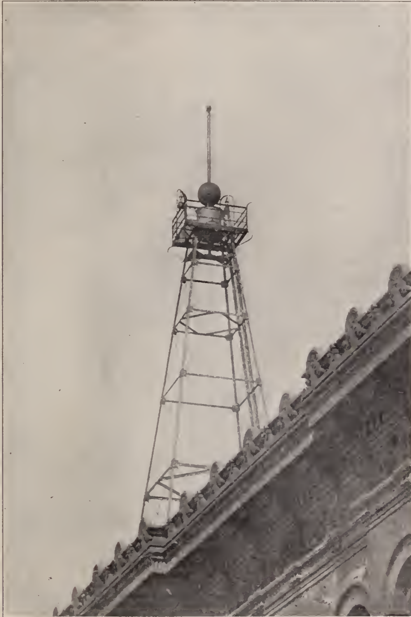
TIME BALL ON TOP OF WESTERN UNION BUILDING, DEY ST. AND BROADWAY.
