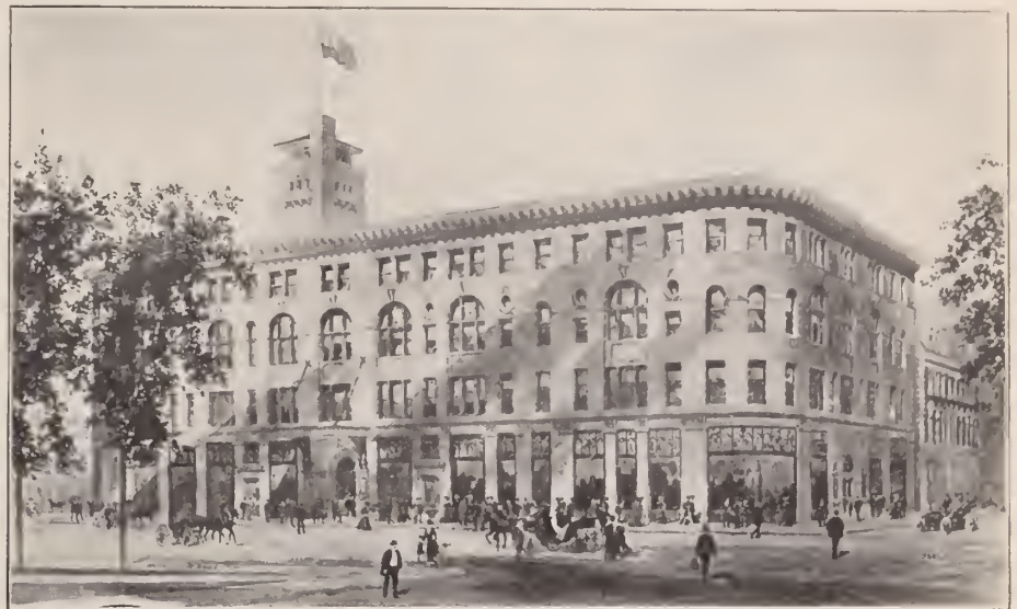
THE NEW ESTABLISHMENT OF HENRY BIRKS & SONS, MONTREAL, CAN., AS IT WILL APPEAR WHEN COMPLETED.
