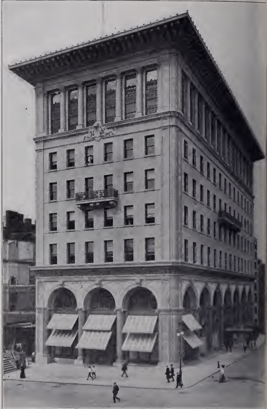
EXTERIOR OF THE NEW BUILDING OF THE GORHAM MFG. CO.
