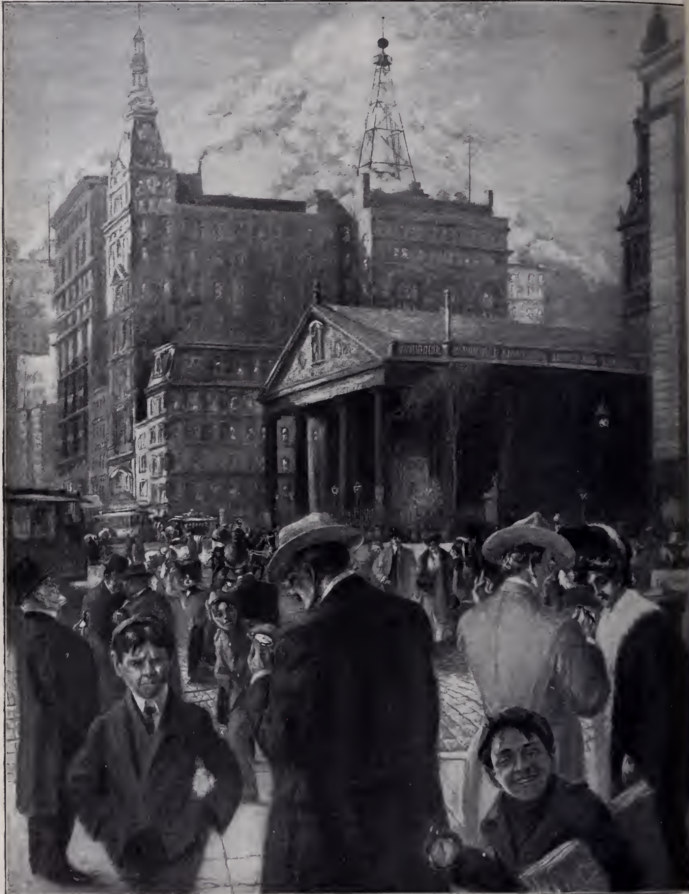
Every day the Time-Ball on the Western Union Building, opposite old St. Paul's, Broadway New York, is dropped at exactly 12 noon, recording Washington time.
