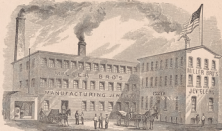
Manufactory, 47, 49 & 51 Franklin Street, JAMES W. MILLER. Newark, N.J. ISAAC M. MILLER.
