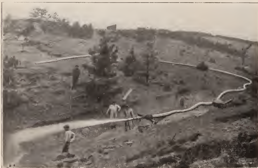
HYDRAULIC MINING FOR SAPPHIRES AT YOGO.
