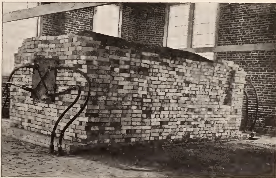
ONE OF THE NEW FURNACES IN OPERATION.
