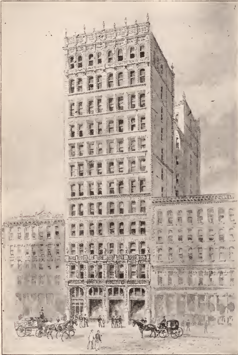
HOW THE FAHYS BUILDING WILL LOOK WHEN FINISHED.
