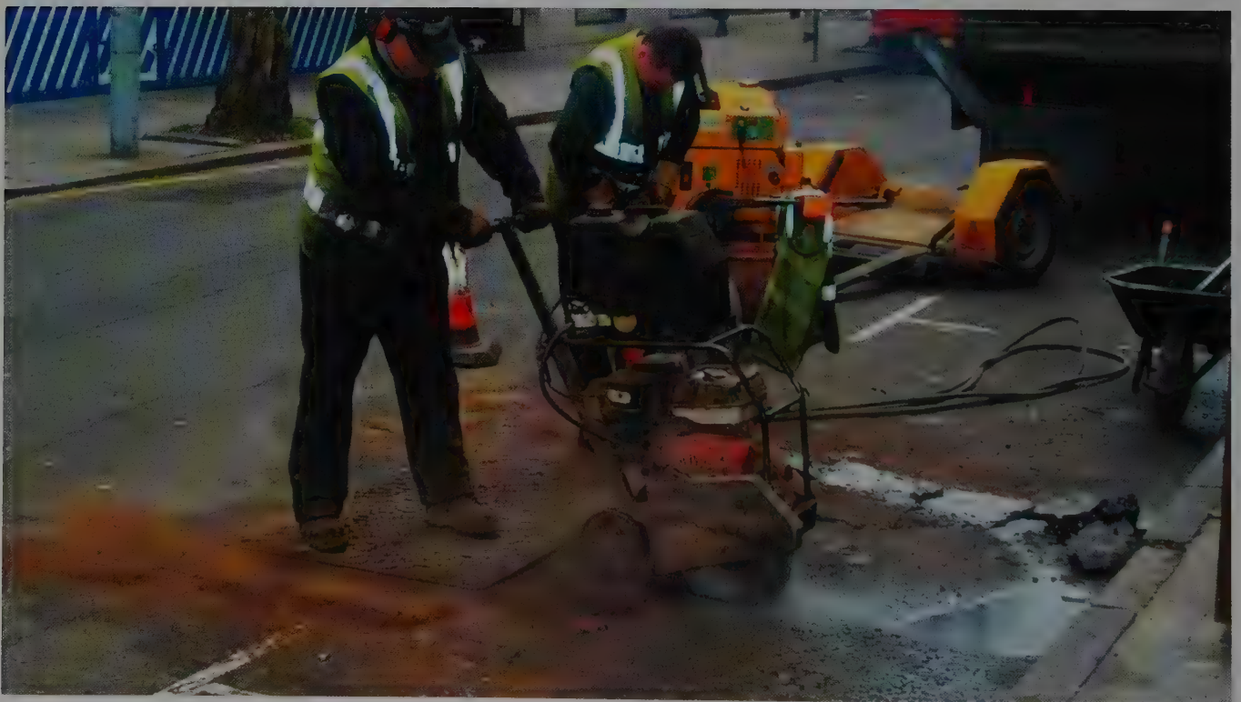
20 A diamond saw being used to 'slice' through a road.
