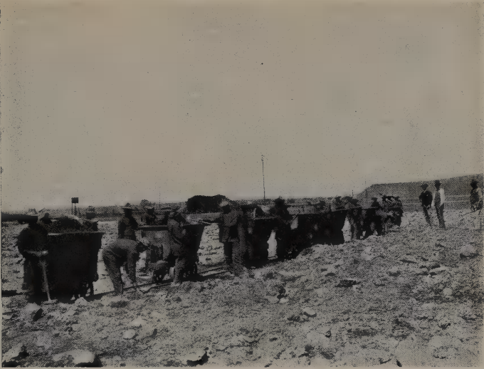
1. LOADING IT ON TO THE FLOORS
